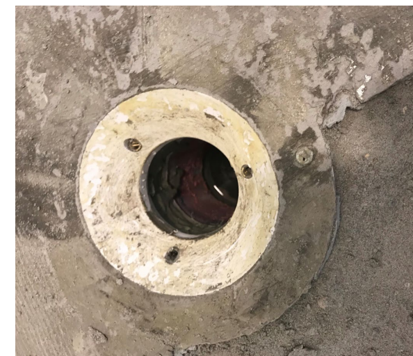
Substrate contaminated with old adhesive residue
