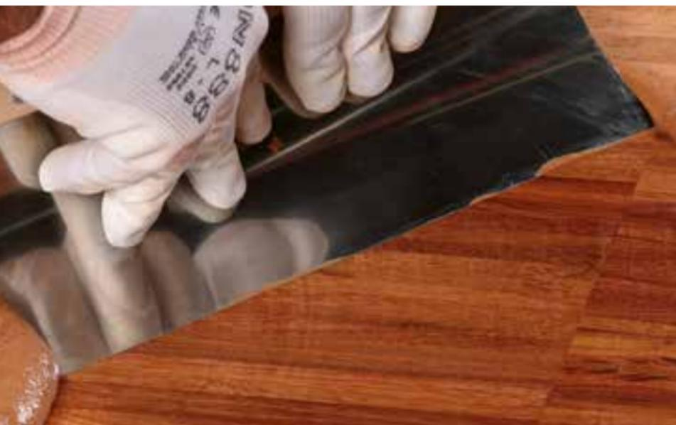
**Solvent and NMP-free odourless water-based binder mixed with wood flour filler for grouting wooden flooring. Suitable for Ultracoat and Ultracoat Oil water-based varnishing cycles.**
