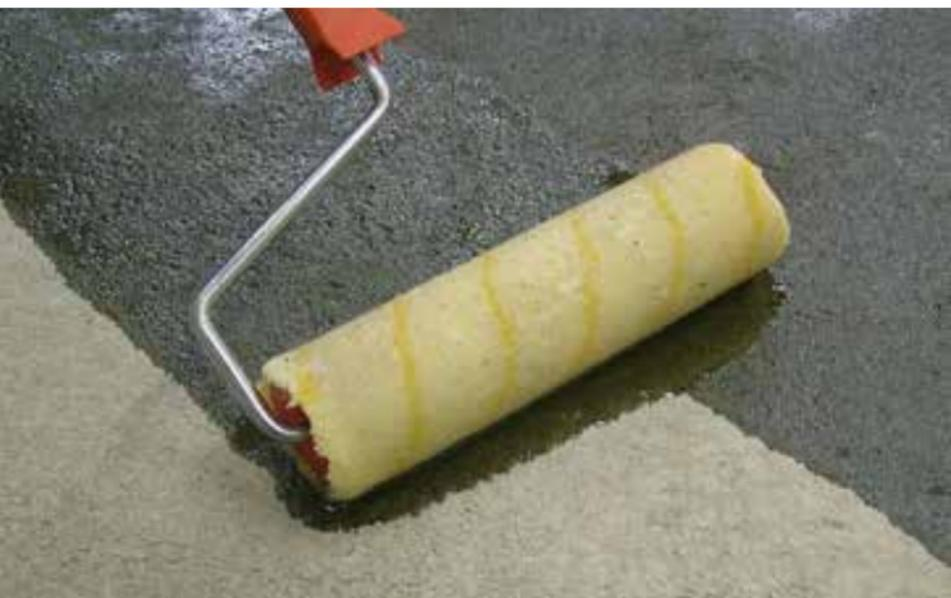
**One-component solvent-free moisture-hardening polyurethane primer with very low emission of volatile organic compounds (VOC) for consolidating and waterproofing cementitious screeds.**
