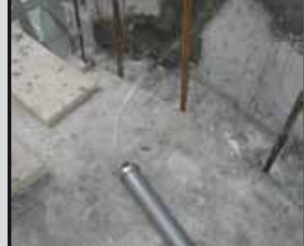
photo 18 Anchor points made using EPOJET
