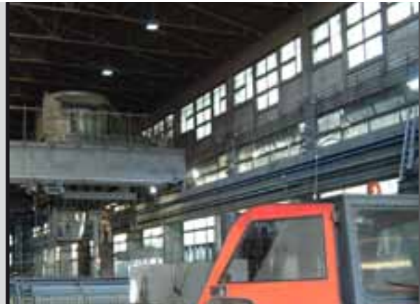
photo 2 Guide rails of an overhead crane
