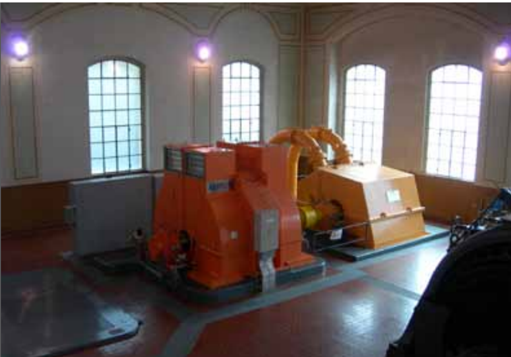
photo 1 Anchorage of a turbine in a power station
