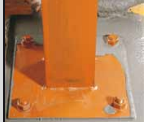
photo 13 Anchoring a metal footing plate with MAPEFILL
