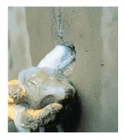
CONSUMPTION 1.8 kg/dm³ of cavity to be filled
