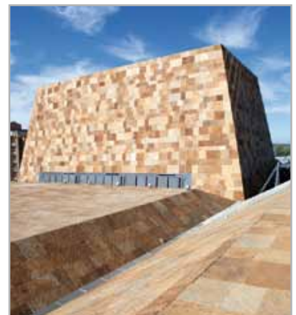
Fig. 4.3 - Example of installation of natural stone on façade - "La Llotja" Congress Centre, Lleida - Spain
