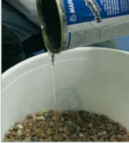
Fig. 5.6 - Mixing of drainage mortar and grout for paved floors with MAPEDRAIN MORTAR
