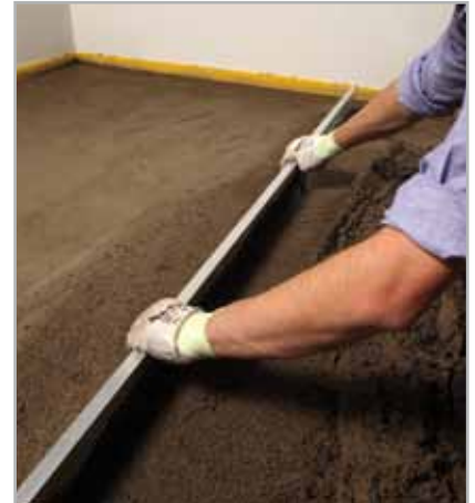
Fig. 3.4 - Using a straight-edge on the screed
