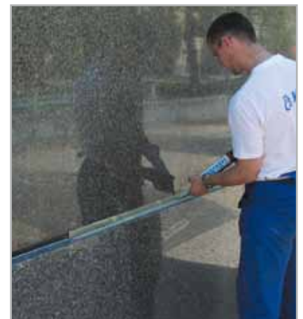
Fig. 4.12 - Sealing joint on façade with MAPESIL LM
