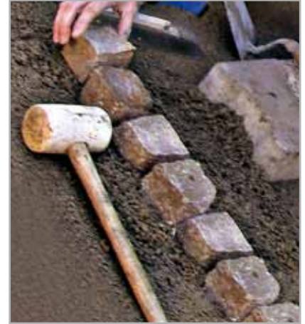
Fig. 5.3 - Installation of porphyry cubes with MAPEDRAIN MORTAR
