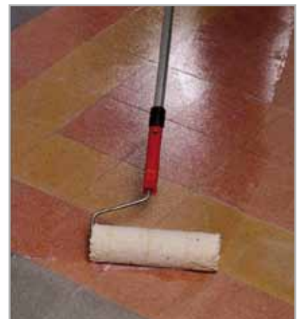
Fig. 3.6 - Applying a primer as bonding promoter
