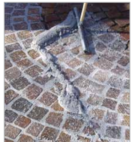
Fig. 5.5 - Application of MAPEDRAIN 3K GROUT
