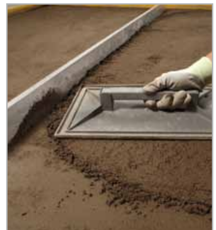
Fig. 3.5 - Floating the screed's surface
