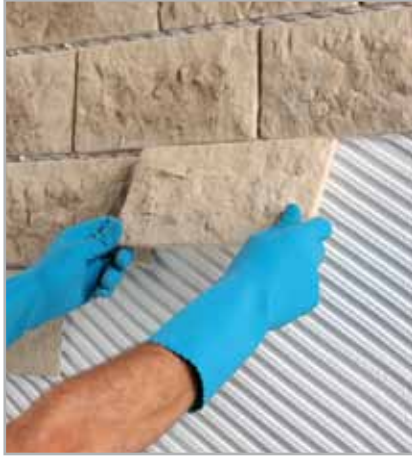
Fig. 5.1 - Laying recomposed decorative elements with FIX & GROUT BRICK
