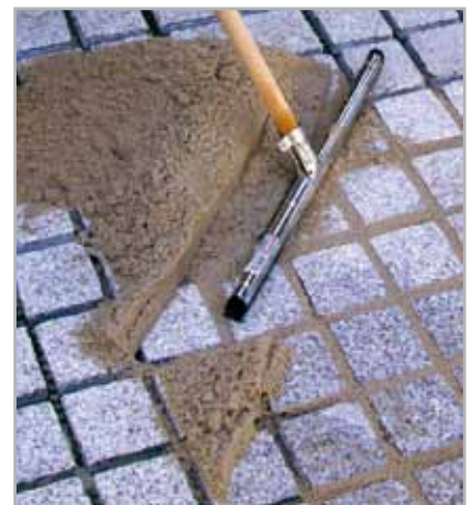
Fig. 5.4 - Application of MAPEDRAIN 1K GROUT
