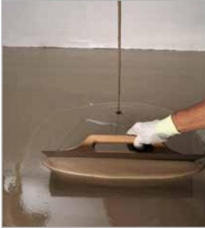
Fig. 3.7 - Levelling a cementitious screed with ULTRAPLAN
