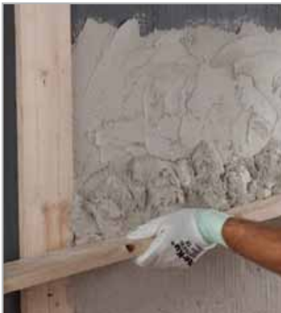
Fig. 3.8 - Evening out a concrete wall with NIVOPLAN+PLANICRETE
