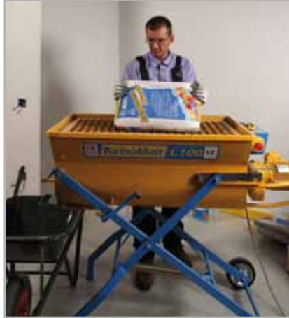
Fig. 3.1 - Mixing MAPECEM PRONTO screed
