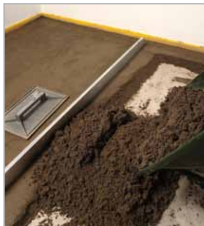
Fig. 3.3 - Carrying out a MAPECEM PRONTO screed
