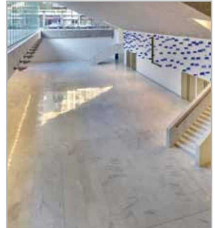
Fig. 4.4 - Example of installation of White Carrara marble with GRANIRAPID white – University Bocconi, Milan – Italy
