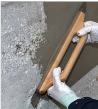
Fig. 3.9 - Evening out a wall with PLANITOP FAST 330
