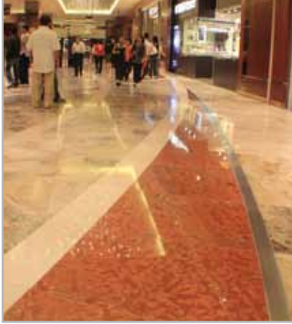
Fig. 4.7 - Example of installation of marble with ELASTORAPID – Marina Bay Sands Resort – Singapore
