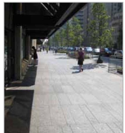
Fig. 4.5 - Example of installation of granite with GRANIRAPID – Bloor Street, Toronto – Canada
