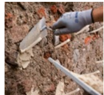
Fastening the small rubber injection tubes in place
