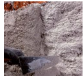
Application of dehumidifying render
