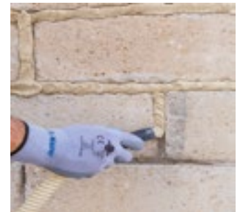
Building stone masonry
