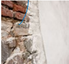
Dehumidifying render mixed on site
