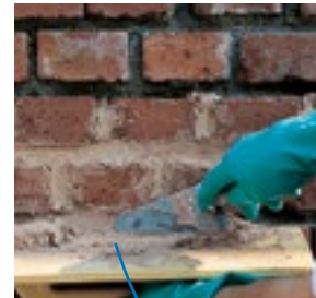
Pointing between brickwork
