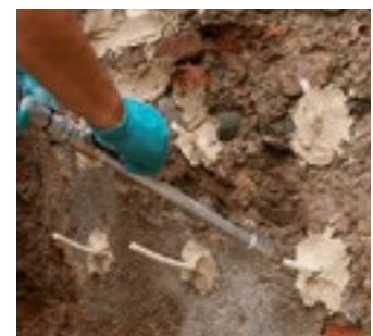
Injecting Mape-Antique I-15
