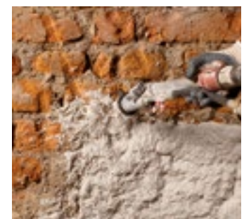
Application of a scratch-coat layer with a rendering machine
