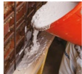
Pouring the mortar made from Mape-Antique Colabile and Gravel 6-10
