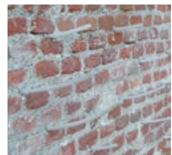
Consolidation of a brick parapet wall
