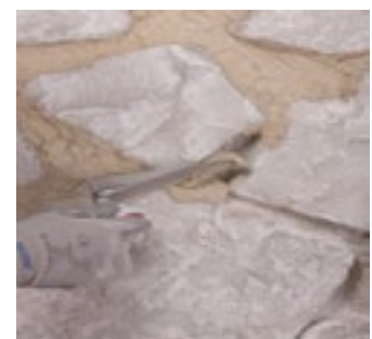
Pointing “exposed” masonry
