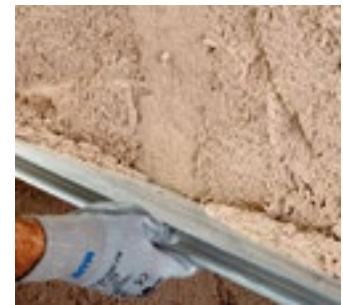
Compacting the dehumidifying render with a straightedge
