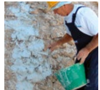
Application of a scratch-coat layer by trowel
