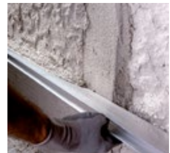
Compacting the dehumidifying render with a straightedge
