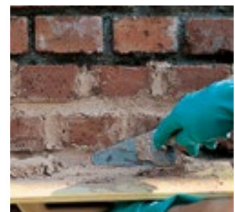
Pointing between brickwork
