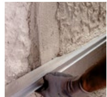
Compacting the dehumidifying render with a straightedge
