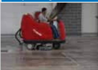
Going over the surface with a polishing machine
