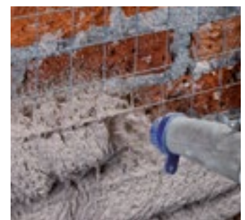
Application of the “structural” render with a rendering machine
