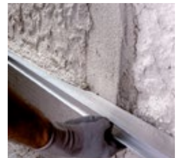
Compacting the dehumidifying render with a straightedge
