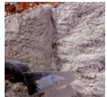
Application of dehumidifying render
