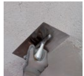
Application of fine texture skimming mortar
