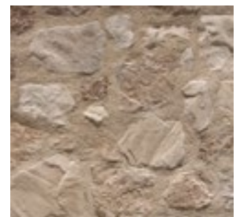
Reconstruction of a stone facing wall
