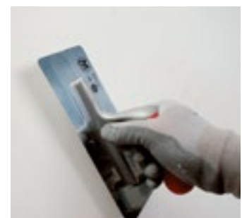
Smoothing over the surface with a flat metal trowel
