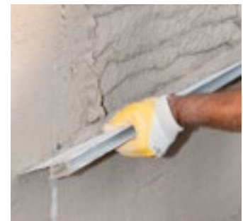
Compacting the transpirant render with a straightedge
