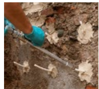
Injecting Mape-Antique I-15
