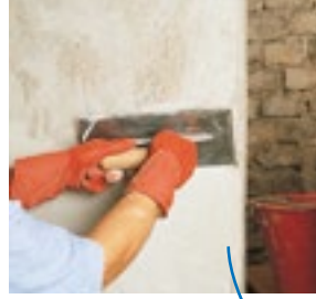
Spreading a transpirant, smooth texture skim coat
