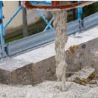
Casting mortar into formwork
