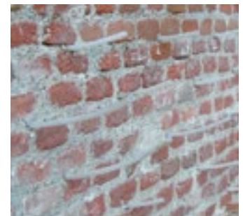
Consolidation of a brick parapet wall
