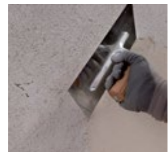
Application of coarse texture skimming mortar
