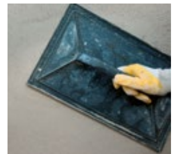
Levelling off the transpirant render
