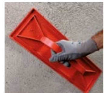
Levelling off the dehumidifying render
