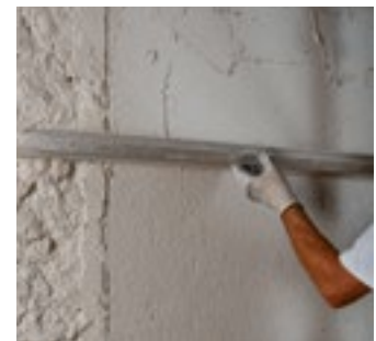
Compacting the dehumidifying render with a straightedge
