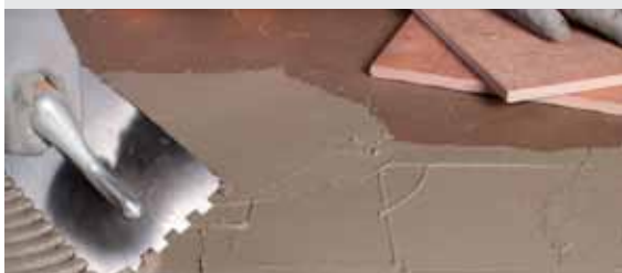
Bonding tiles with Granirapid
