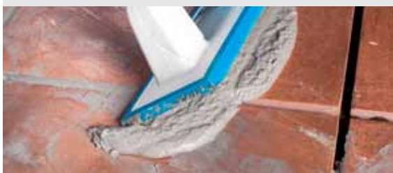
Grouting tiles with Ultracolor Plus
