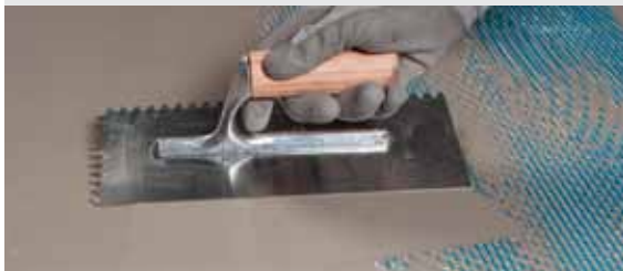
Placing Mapenet 150 on the first layer of Mapelastic Turbo
