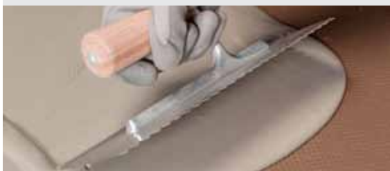
Application of the second layer of Mapelastic Turbo
