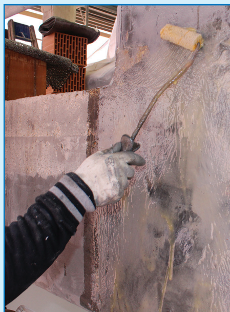
First coat of MapeWrap 31
