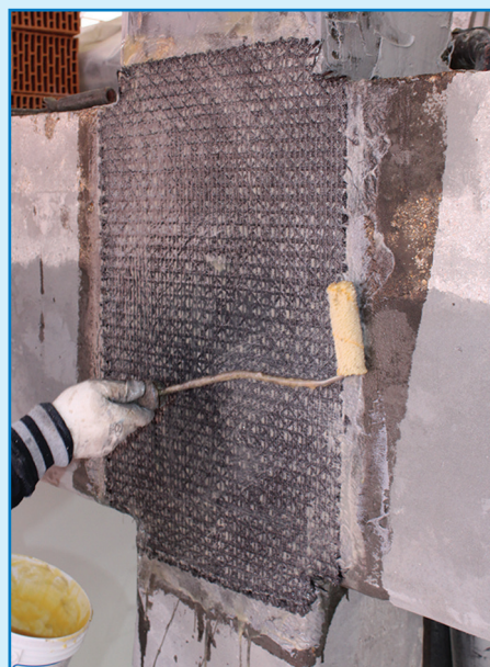
Second coat of MapeWrap 31
