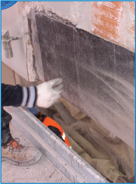
Broadcasting of quartz sand
