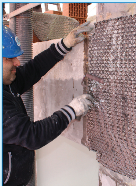
Application of MapeWrap C QUADRI-AX fabric
