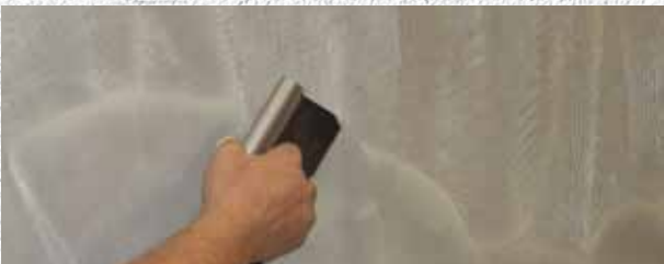
Application of Ultrabond Eco 530 adhesive
