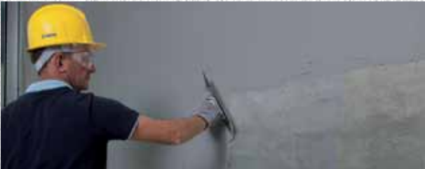
Skimming the wall with Planipatch
