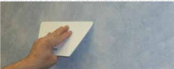
Application of resilient wall covering
