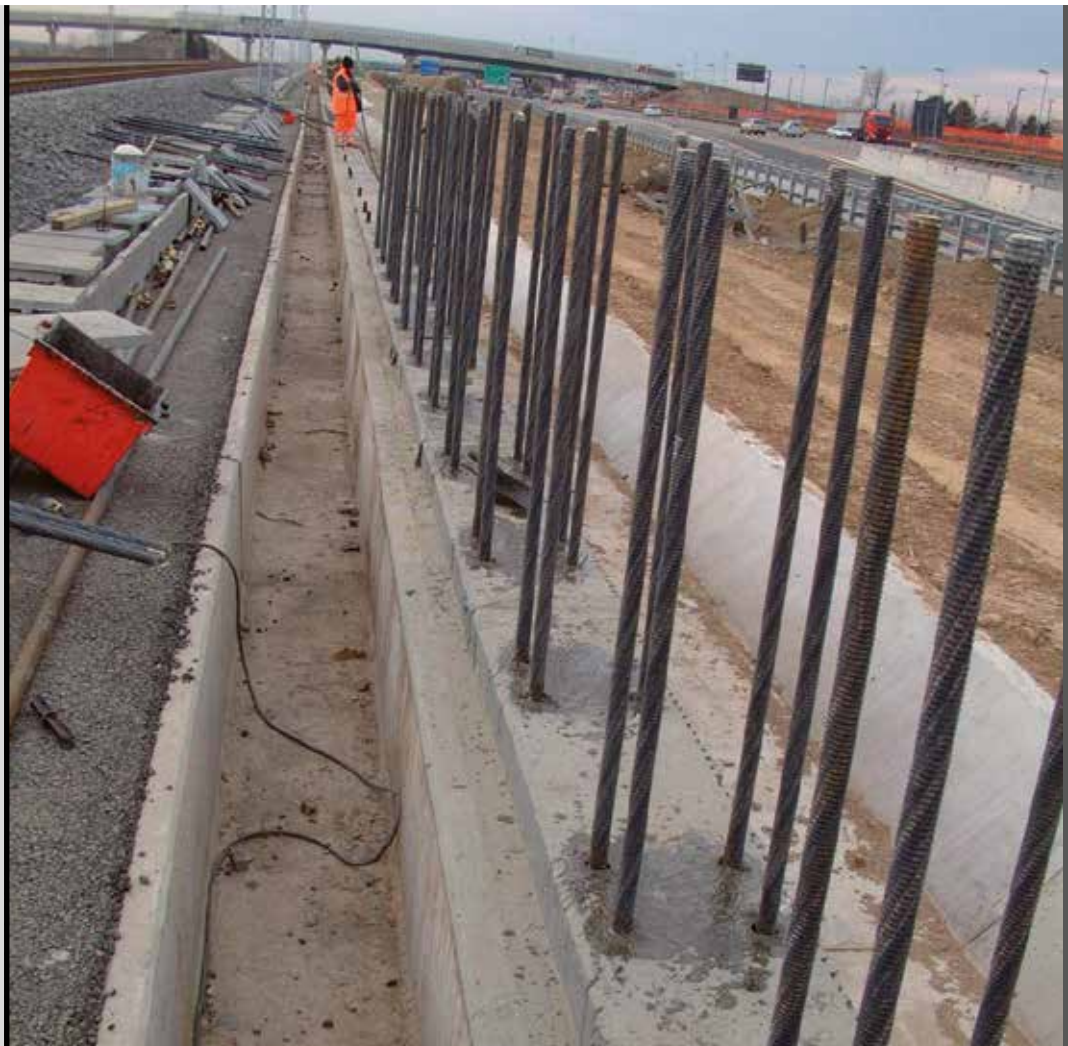
Photo 12 Anchoring steel bars in concrete using PLANIGROUT 300
