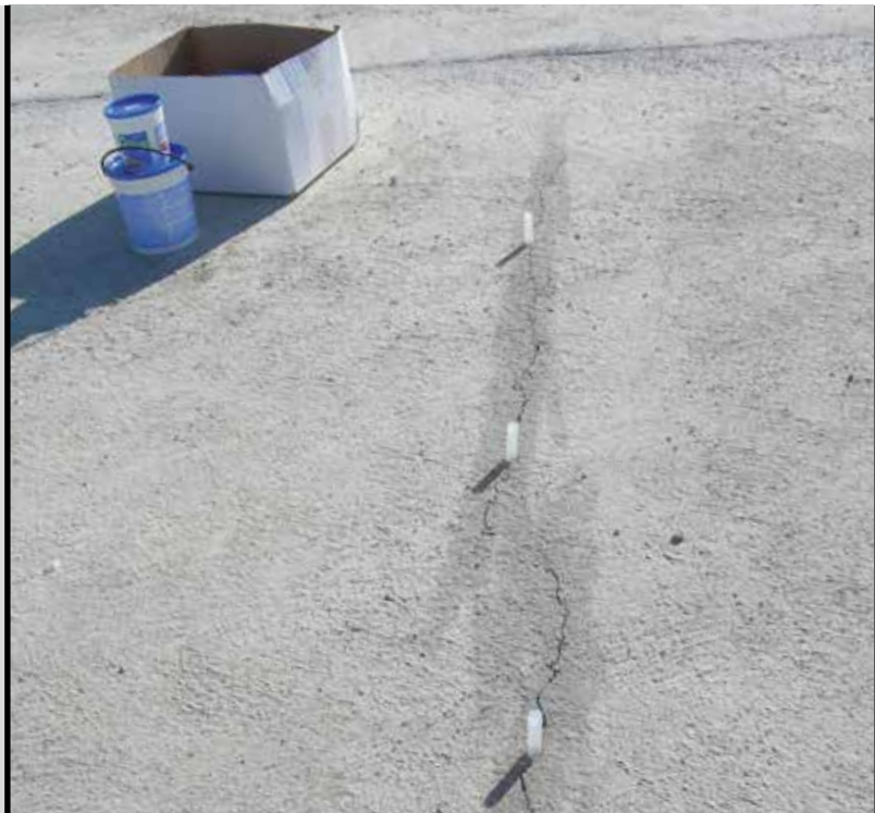
Photo 11 Injecting EPOJET in a cracked concrete slab
