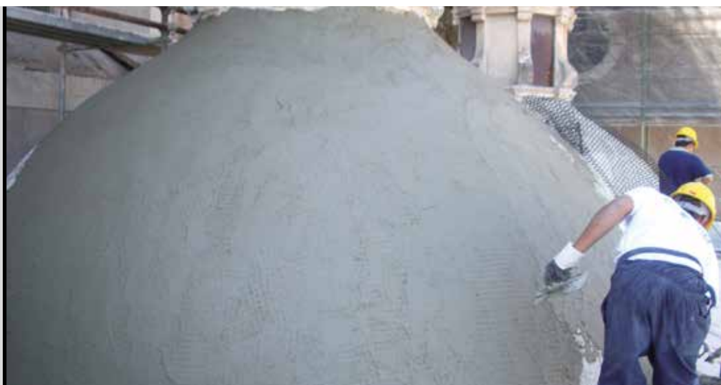
Photo 5 Strengthening of a concrete structure with PLANITOP HDM + MAPEGRID G220 , non-structural class R2 mortar
