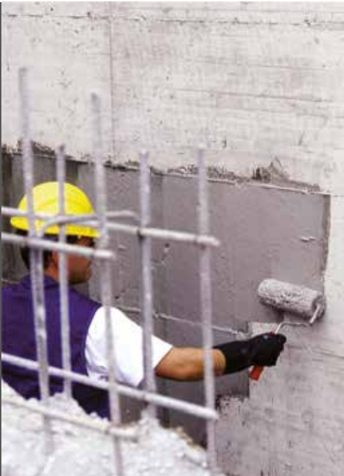
photo 17 MAPELASTIC SMART applied with a roller
