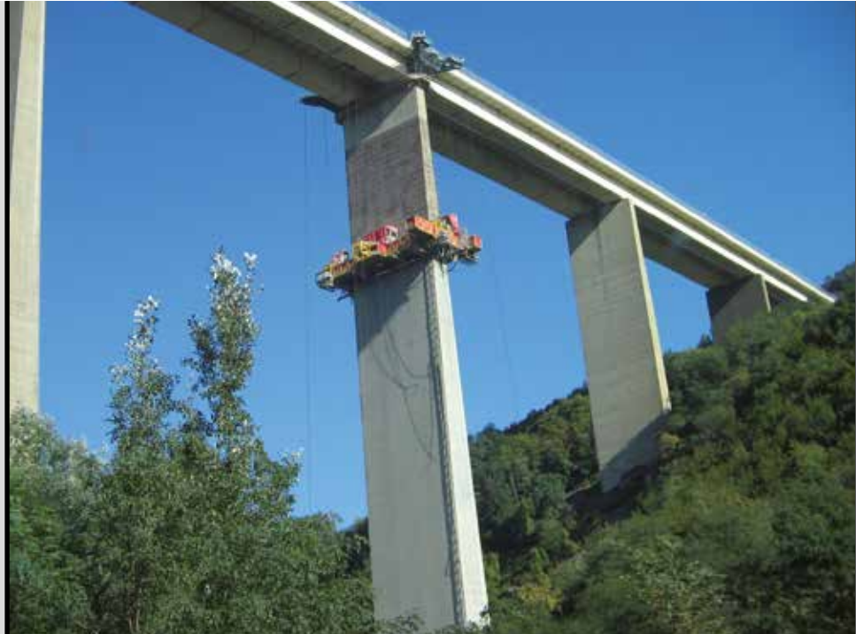
photo 2 Hydro-scarifying operations on a viaduct pile
