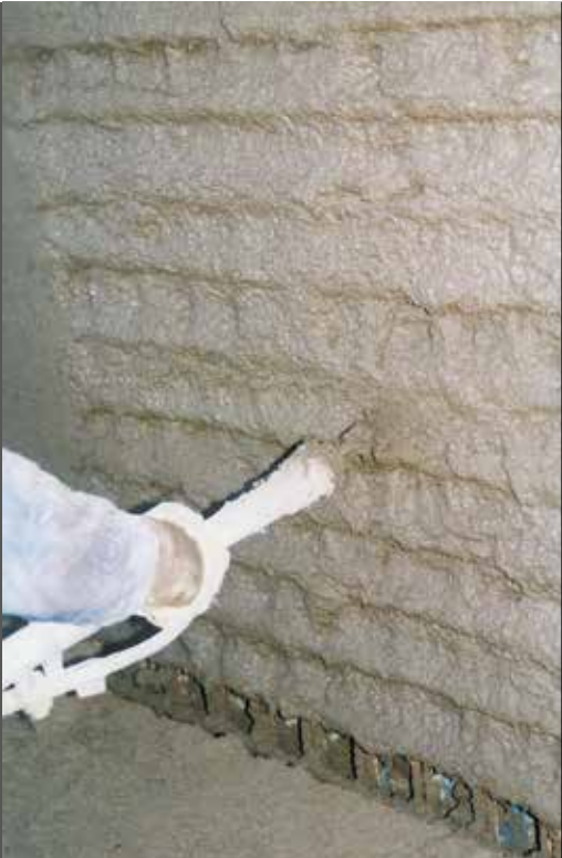
photo 5 MAPEGROUT EASY FLOW applied by spray
