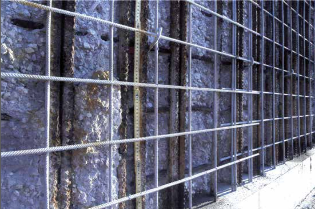
photo 4 Positioning new reinforcement
