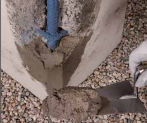
photo 9 Application of MAPEGROUT LM2K
