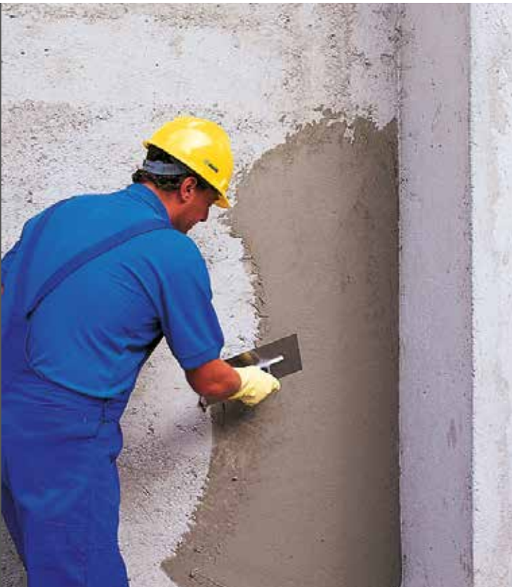
photo 20 Smoothing layer using MONOFINISH
