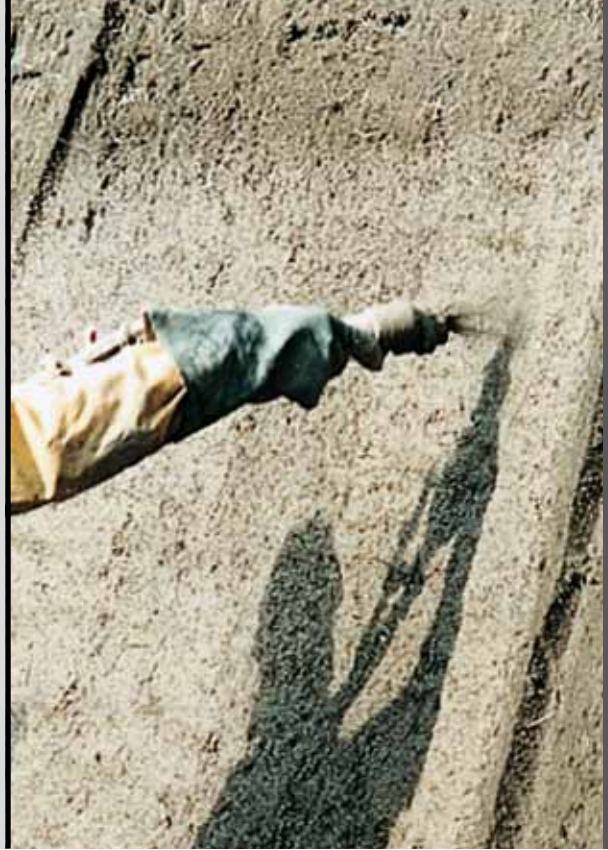
photo 8 Mapegrout FMR applied by spray
