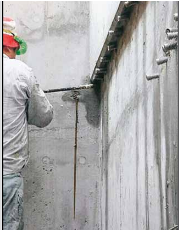
photo 15 Injection of Foamjet F
