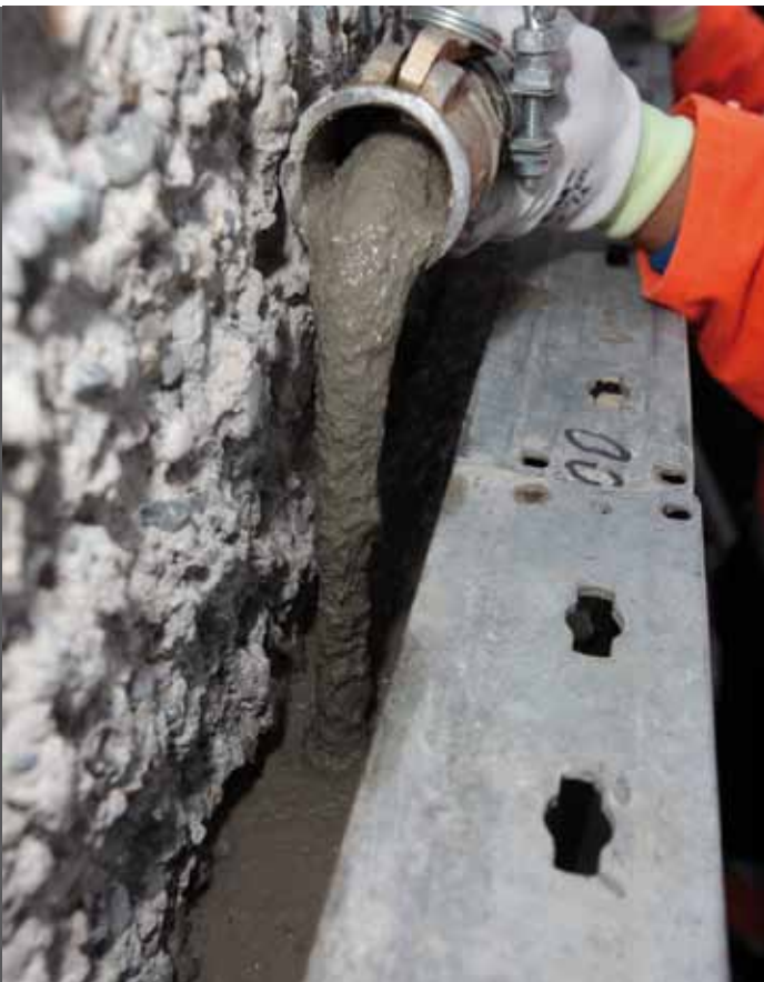
photo 13 Application of Mapegrout Hi-Flow GF
