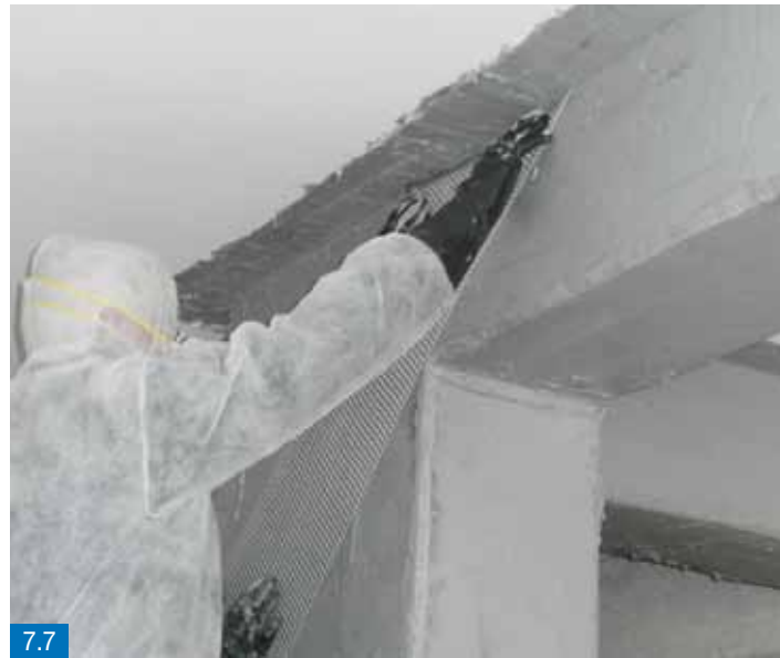
Figures 7.6 and 7.7 - Shear strengthening of a column/beam junction using MAPEWRAP S FABRIC
