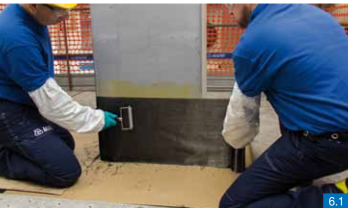
Figure 6.1 - Confinement of a reinforced concrete panel using uniaxial carbon fibre (MAPEWRAP C)
