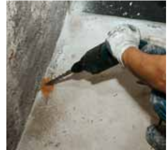
Drilling the holes
