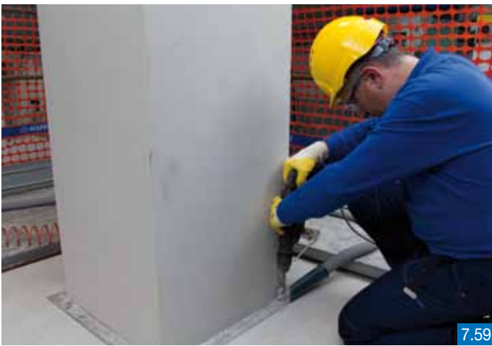
Figure 7.60 - Priming the surfaces of the pillar with MAPEWRAP PRIMER 1
