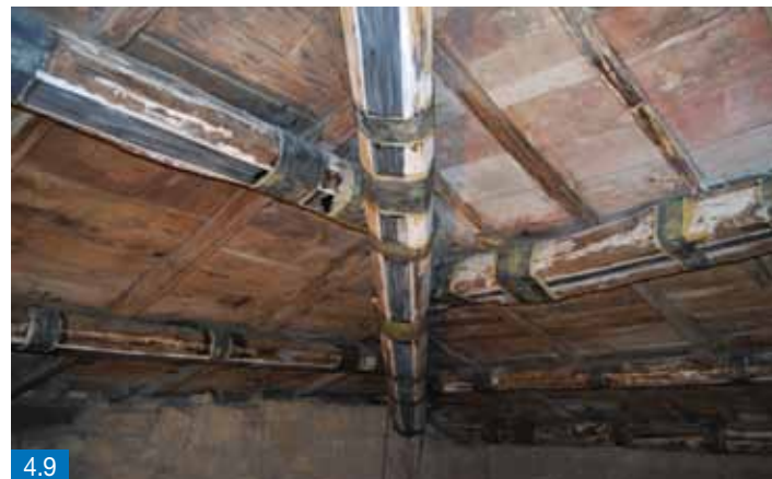
Figures 4.8 and 4.9 - Strengthening of wooden beams using CARBOPLATE plates - Palazzo Farnese, Italy
