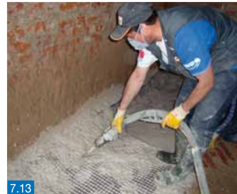
Figures 7.11, 7.12, 7.13, 7.14, 7.15 and 7.16 - Strengthening the outer face of masonry vaults using PLANITOP HDM and MAPEGRID G 220 - Palazzo Sforza, Milan (Italy)
