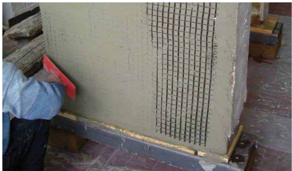
Figure 5.4 - A panel with a strengthening system applied: MAPEGRID G220 + PLANITOP HDM
