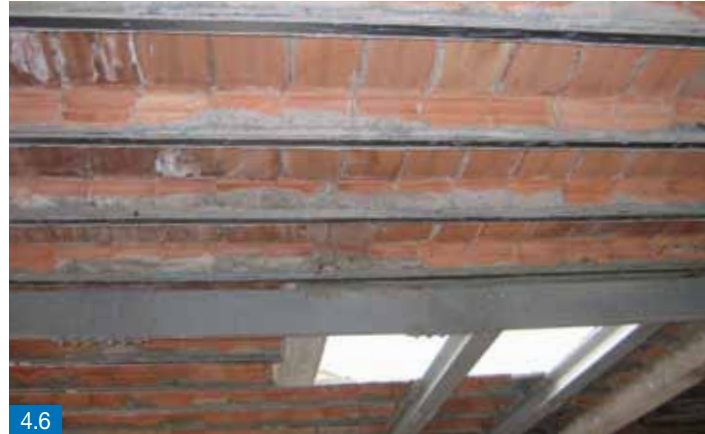
Figure 4.5 - Flexural strengthening of joists using MAPEWRAP C UNI-AX fabric
