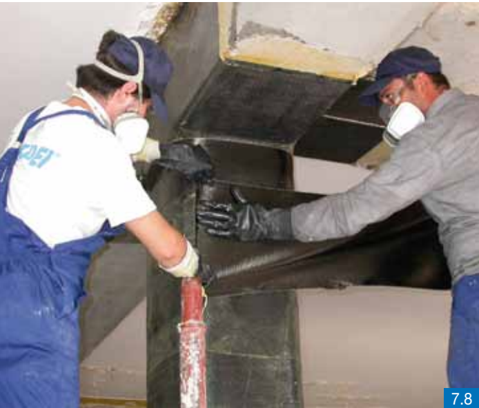
Figures 7.8, 7.9 and 7.10 - Seismic upgrading of beam-column hinge zones using MAPEWRAP fabrics
