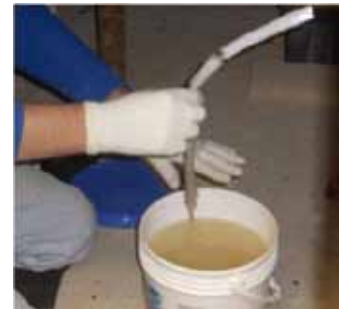
Impregnating a portion of MAPEWRAP FIOCCO
