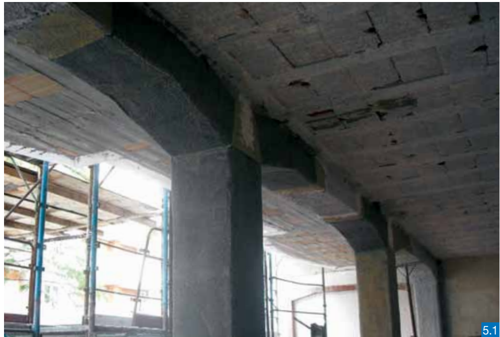
Figure 5.1 - Shear strengthening of a reinforced concrete beam
