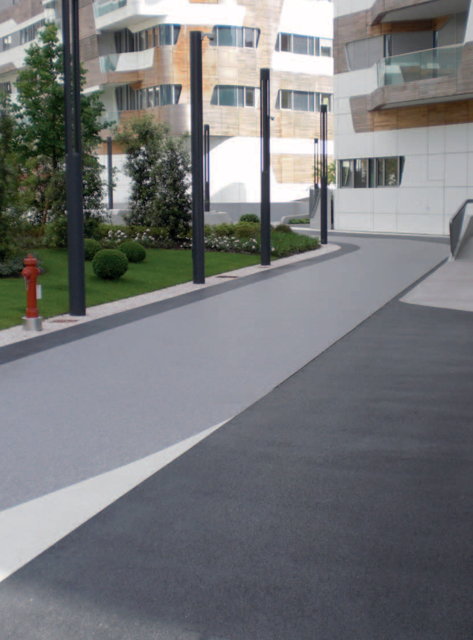
Pathways running between the houses - City Life - Milan - Products used in the system: MAPEFLOOR URBAN SYSTEM
