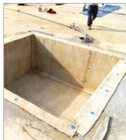
Fig. 7.5b – Lift well lined with MAPEPROOF
