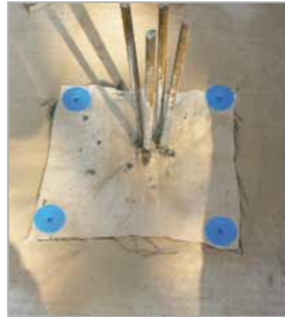
Fig. 7.26 – A piece of sheet nailed to the substrate
