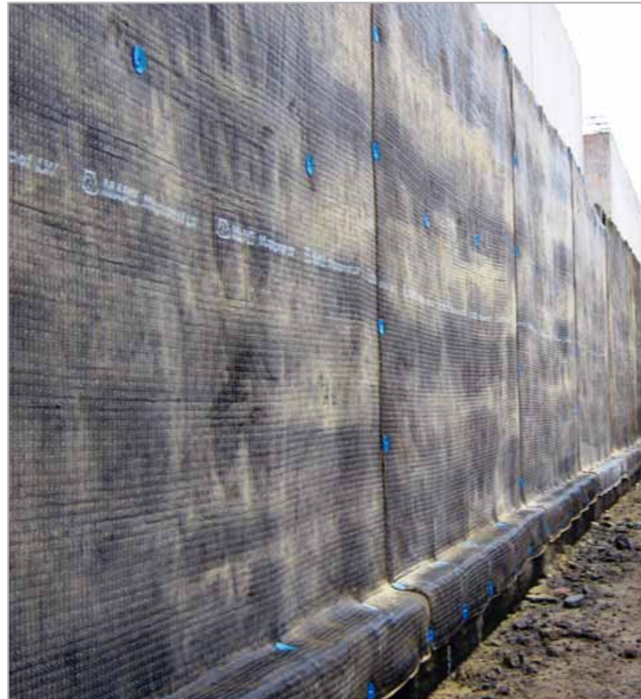
Fig. 5.3 – An example of MAPEPROOF applied after casting
