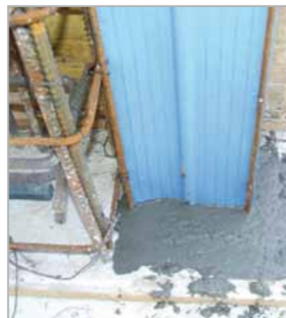
Fig. 7.56e – Repairing foundations with MAPEGROUT COLABILE
