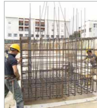
Fig. 7.5c – Positioning the steel reinforcement
