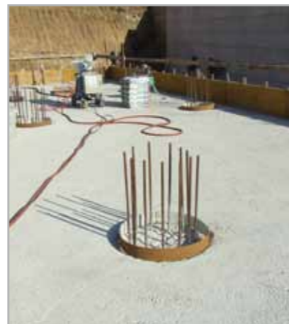
Fig. 7.16 - Metallic cylindrical mould in place before casting MAPEGROUT HI-FLOW
