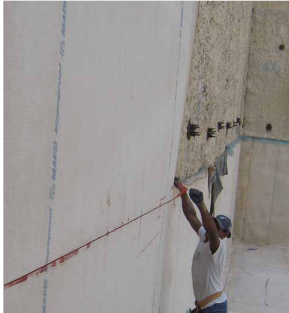
Fig. 7.38 – Application of MAPEPROOF on the lower part of diaphragms
