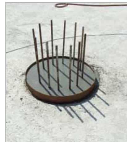
Fig. 7.17 - The head of a pile rebuilt with MAPEGROUT HI-FLOW
