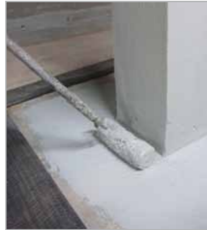
Fig. 8.6b - MAPELASTIC FOUNDATION is also applied also on the pillars
