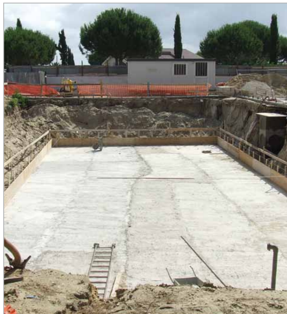
Fig. 4.1 – Stripped ground without confinement
