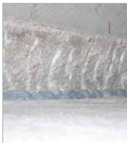
Fig. 8.1c - Construction joint sealed with MAPEPROOF SWELL
