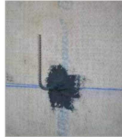
Fig. 7.69 - Grouting metallic connectors with MAPEPROOF MASTIC
