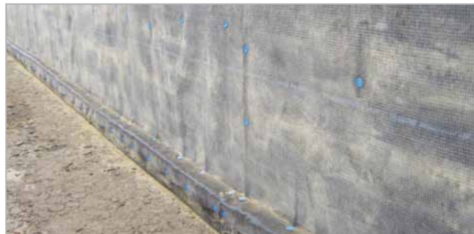
Fig. 7.45b – A vertical wall waterproofed with MAPEPROOF after casting
