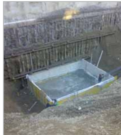
Fig. 7.4 – Waterproofing the base of a jib crane with MAPEPROOF bentonite sheets
