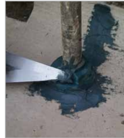
Fig. 7.60e - Further grouting with MAPEPROOF MASTIC
