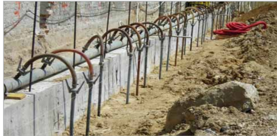
Fig. 3.4 – Flexible hoses used to connect wellpoints to an intake manifold
