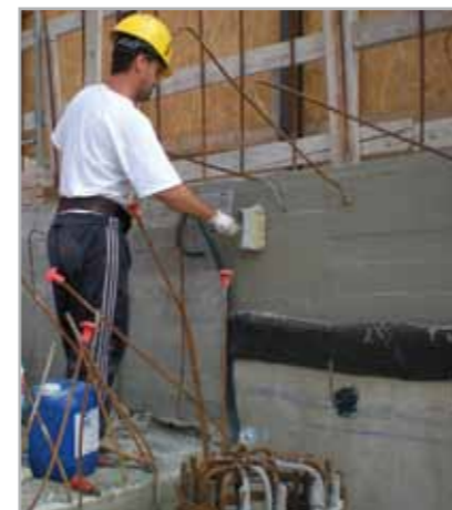
Fig. 7.70 - Application of MAPELASTIC FOUNDATION on the topping beams on the bulkhead
