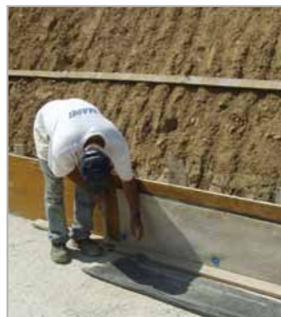
Fig. 7.10 – Nailing MAPEPROOF to wooden formwork
