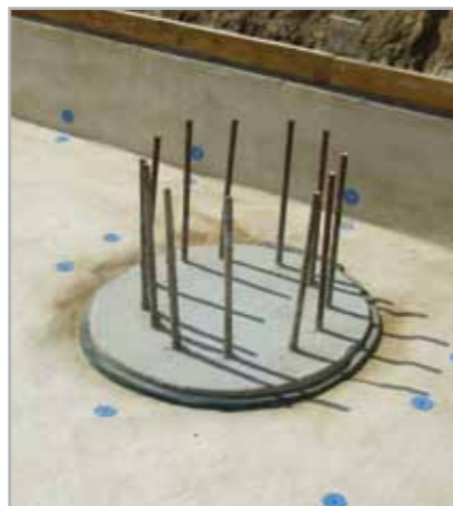
Fig. 7.21 - Application of IDROSTOP B25 around the head of a pile
