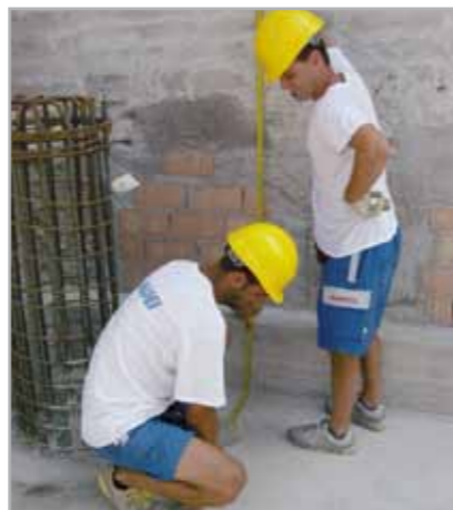
Fig. 7.67 - Taking measurements before cutting MAPEPROOF sheets: start laying the sheets at least 1 m from the bottom of the excavation
