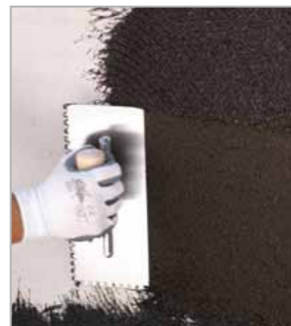
Fig. 7.54 – Application of PLASTIMUL 2K SUPER
