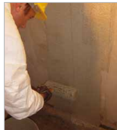
Fig. 8.8e – Application of MAPELASTIC FOUNDATION
