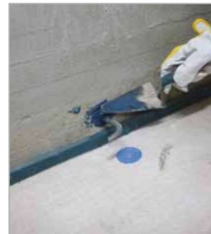
Fig. 8.6f - Grouting the metal connectors with MAPEPROOF MASTIC
