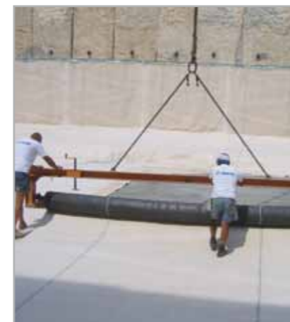
Fig. 7.12 – Laying MAPEPROOF using a metal lifting rig
