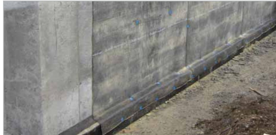
Fig. 7.45A – Nailing MAPEPROOF to the substrate after casting
