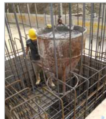
Fig. 7.5d – Casting the foundation pad for a lift well
