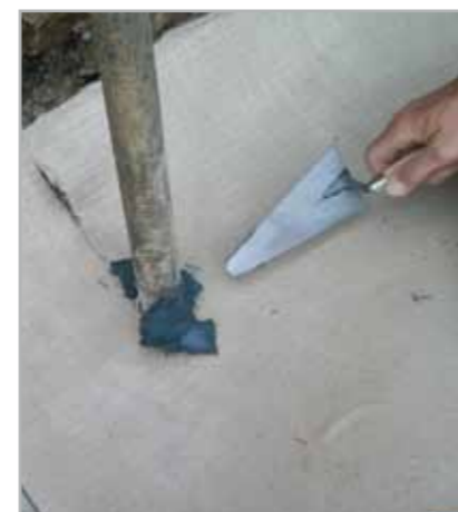
Fig. 7.60b – Application of MAPEPROOF MASTIC on the sheet
