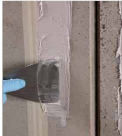
Fig. 7.48b – Spreading on ADESILEX PG4 with a trowel
