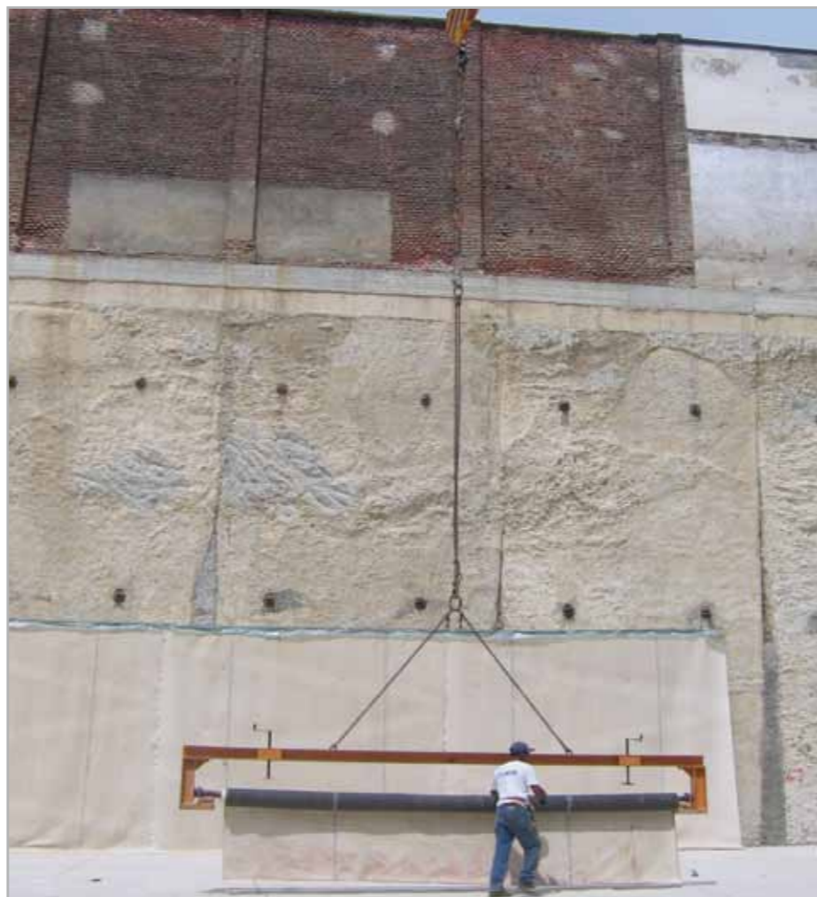
Fig. 7.37 - Laying MAPEPROOF against a diaphragm
