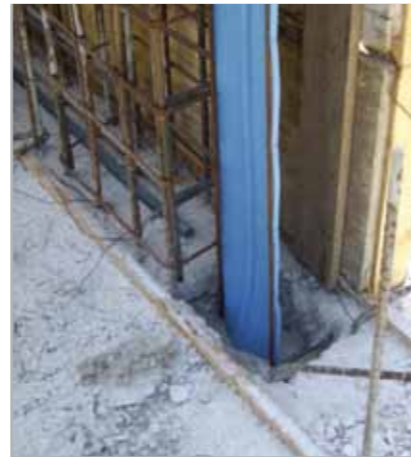
Fig. 7.56c – Positioning and fastening IDROSTOP PVC BI to the steel reinforcement
