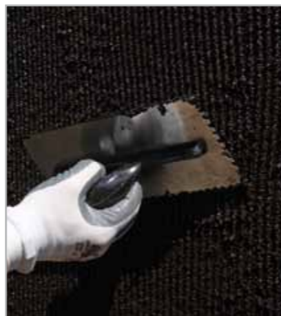
Fig. 7.52 – Application of PLASTIMUL 1K SUPER PLUS
