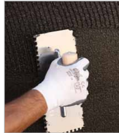
Fig. 7.53 – Application of PLASTIMUL 2K PLUS
