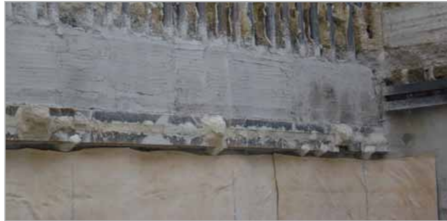
Fig. 7.36 – Bulkhead in micro-piles levelled off with MAPEGROUT T60
