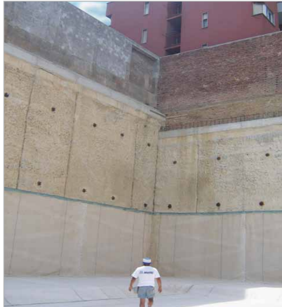
Fig. 4.2 – Stripped ground confined by diaphragms
