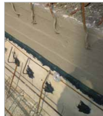
Fig. 7.71 - Sealing a fillet joint between MAPELASTIC FOUNDATION and MAPEPROOF with MAPEPROOF MASTIC and then nailing IDROSTOP B25 in place
