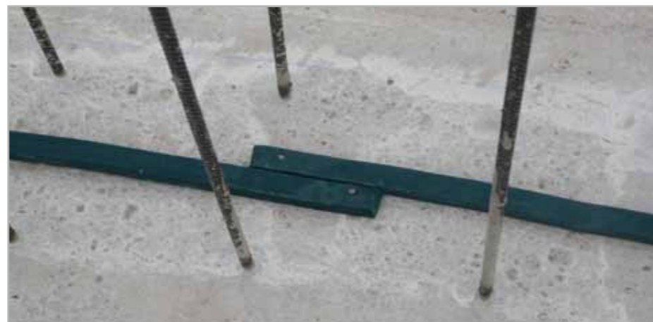
Fig. 7.3 - Joint between the ends of two strips of IDROSTOP B25 by simply laying them alongside each other for at least 6 cm
