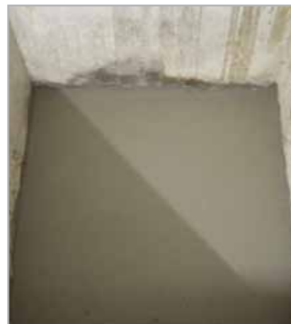
Fig. 8.8b – Screed made from sand, cement and IDROSILEX
