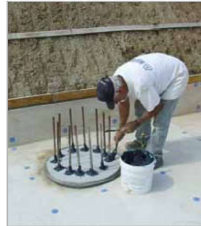
Fig. 7.22 - Grouting the reinforcement in a pile with MAPEPROOF MASTIC
