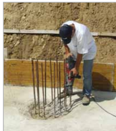
Fig. 7.15 - Cropping the head of a pile
