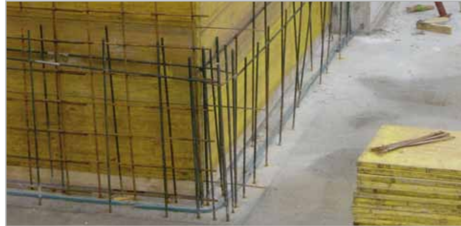
Fig. 7.1 - IDROSTOP B25 applied to seal horizontal and vertical construction joints
