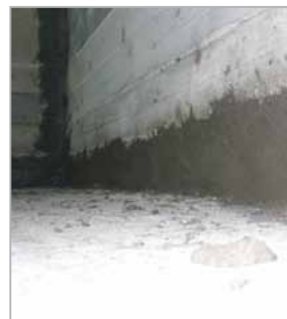
Fig. 8.1e - A sealed, repaired construction joint
