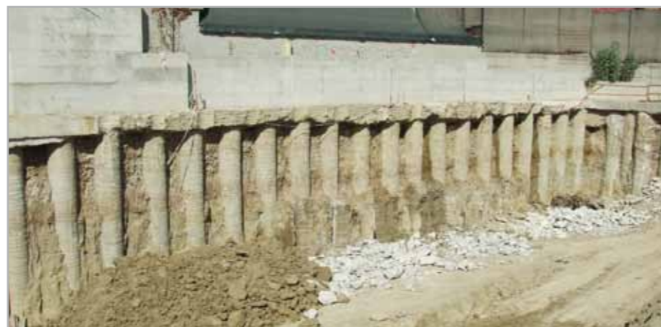
Fig. 4.3 – Stripped ground confined by bored piles
