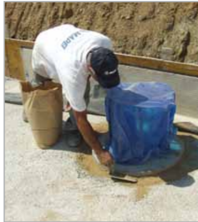
Fig. 7.19 - Sealing around the perimeter of the head of a pile with MAPEPROOF SEAL
