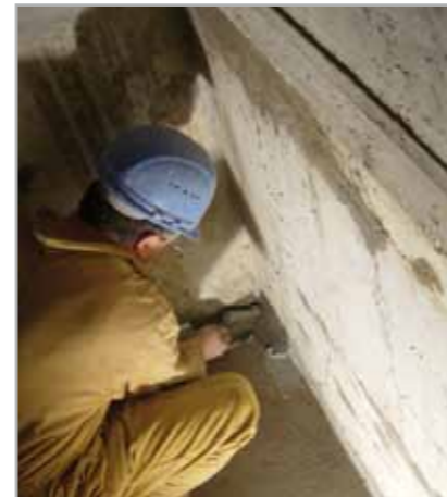
Fig. 8.8d – Making fillets on the EPORIP while still fresh with MAPEGROUT BM
