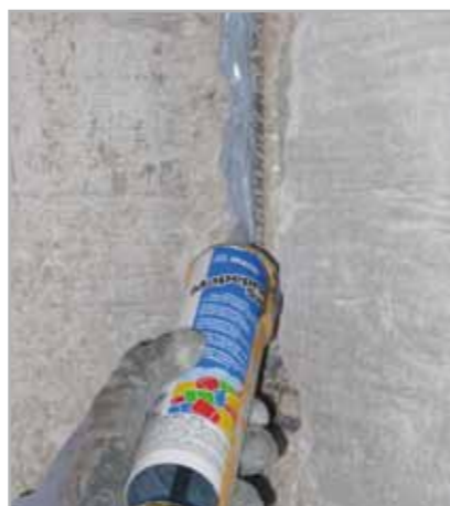
Fig. 8.1b - Extrusion of MAPEPROOF SWELL
