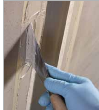
Fig. 7.48d – Spreading on the second layer of ADESILEX PG4 with a trowel
