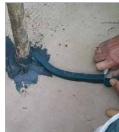
Fig. 7.60c – Laying IDROSTOP B25
