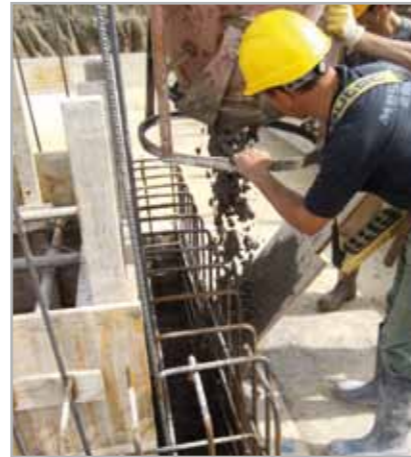
Fig. 7.5f – Casting vertical walls
