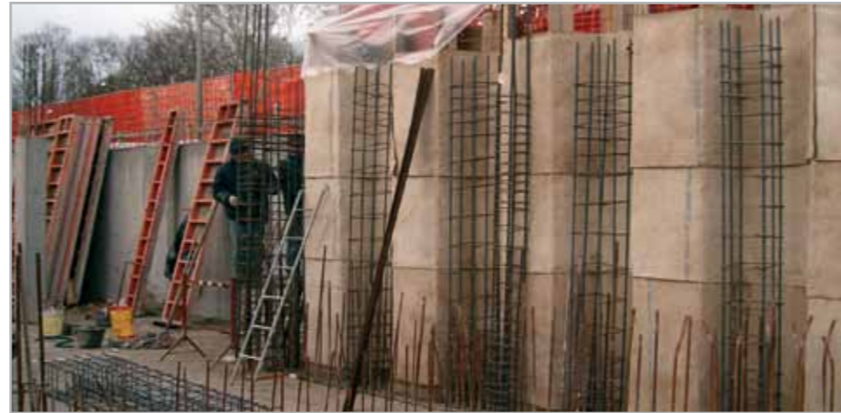
Fig. 7.31 – MAPEPROOF applied directly on sheetpiling
