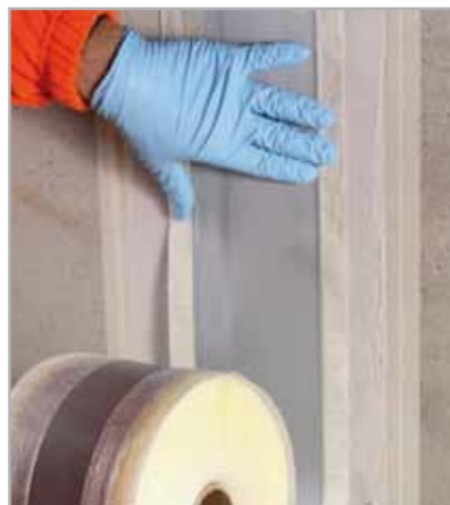
Fig. 7.48c – Positioning MAPEBAND TPE
