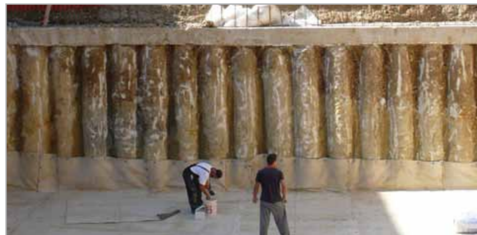
Fig. 7.32 – MAPEPROOF applied directly on a pile bulkhead
