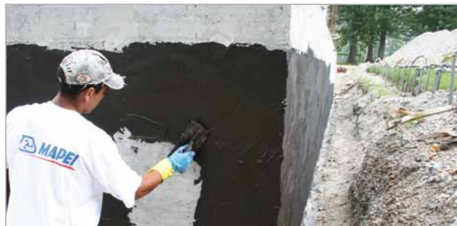
Fig. 7.50 – Using a trowel to apply PLASTIMUL on a vertical retaining wall
