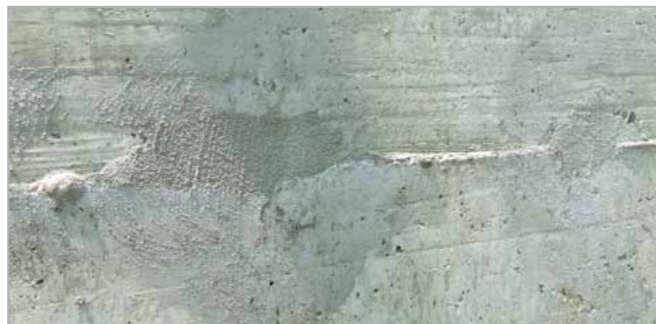
Fig. 7.44 – Levelling off the concrete surface after removing the blades of the formwork
