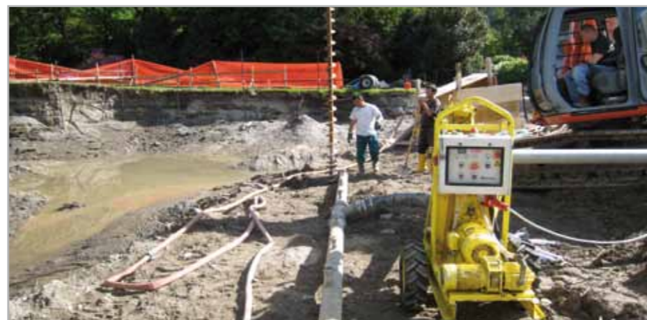
Fig. 3.6 – Drilling operations to insert wellpoints
