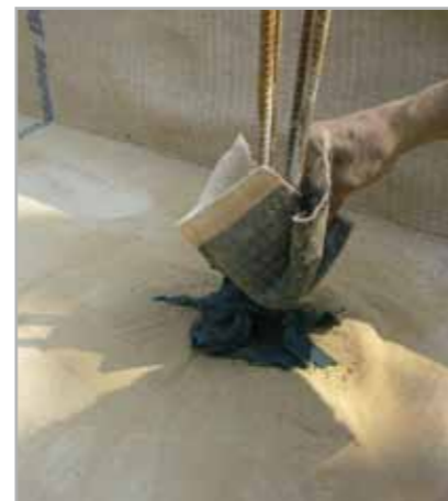
Fig. 7.25 - Localised reinforcement of the waterproofing with a piece of MAPEPROOF grouted with MAPEPROOF MASTIC
