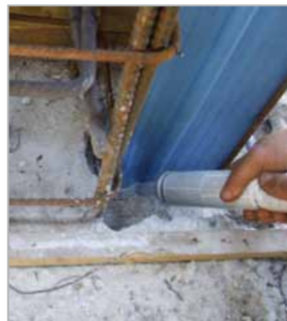
Fig. 7.56d – Sealing with MAPEPROOF SWELL
