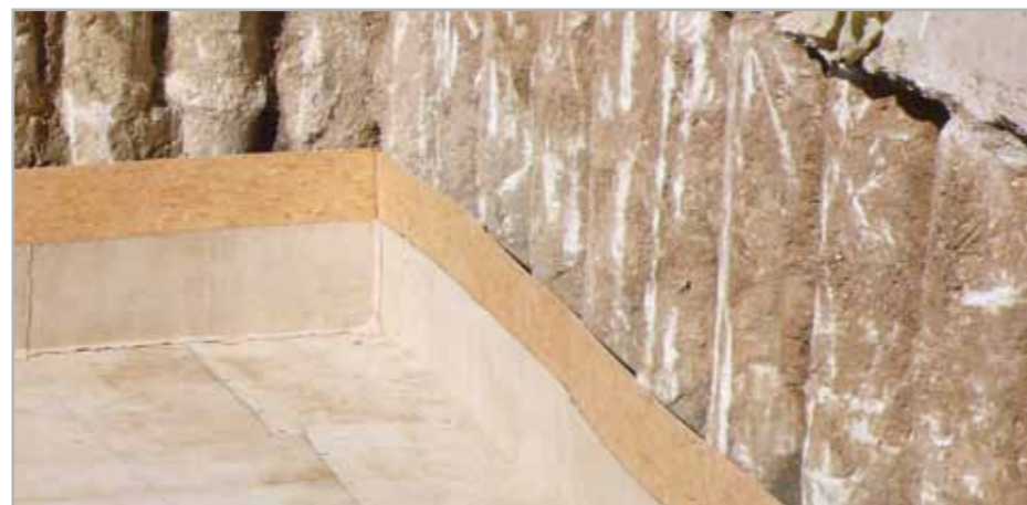
Fig. 7.33 – Application of MAPEPROOF on OSB panels laid against piles
