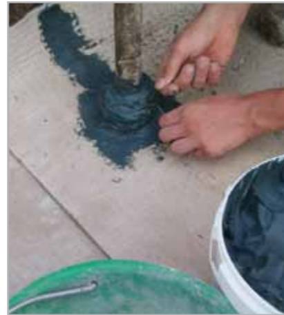
Fig. 7.60d - Fastening IDROSTOP B25 in place with metal wire
