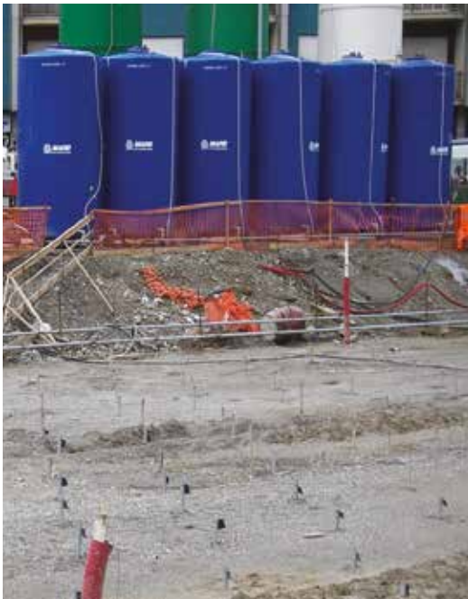
Turin subway: bottom slab waterproofing
