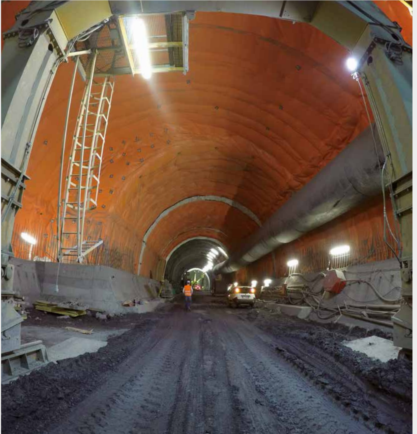
HIGH SPEED RALWAY MILAN-GENOA BASE TUNNEL - Italy
