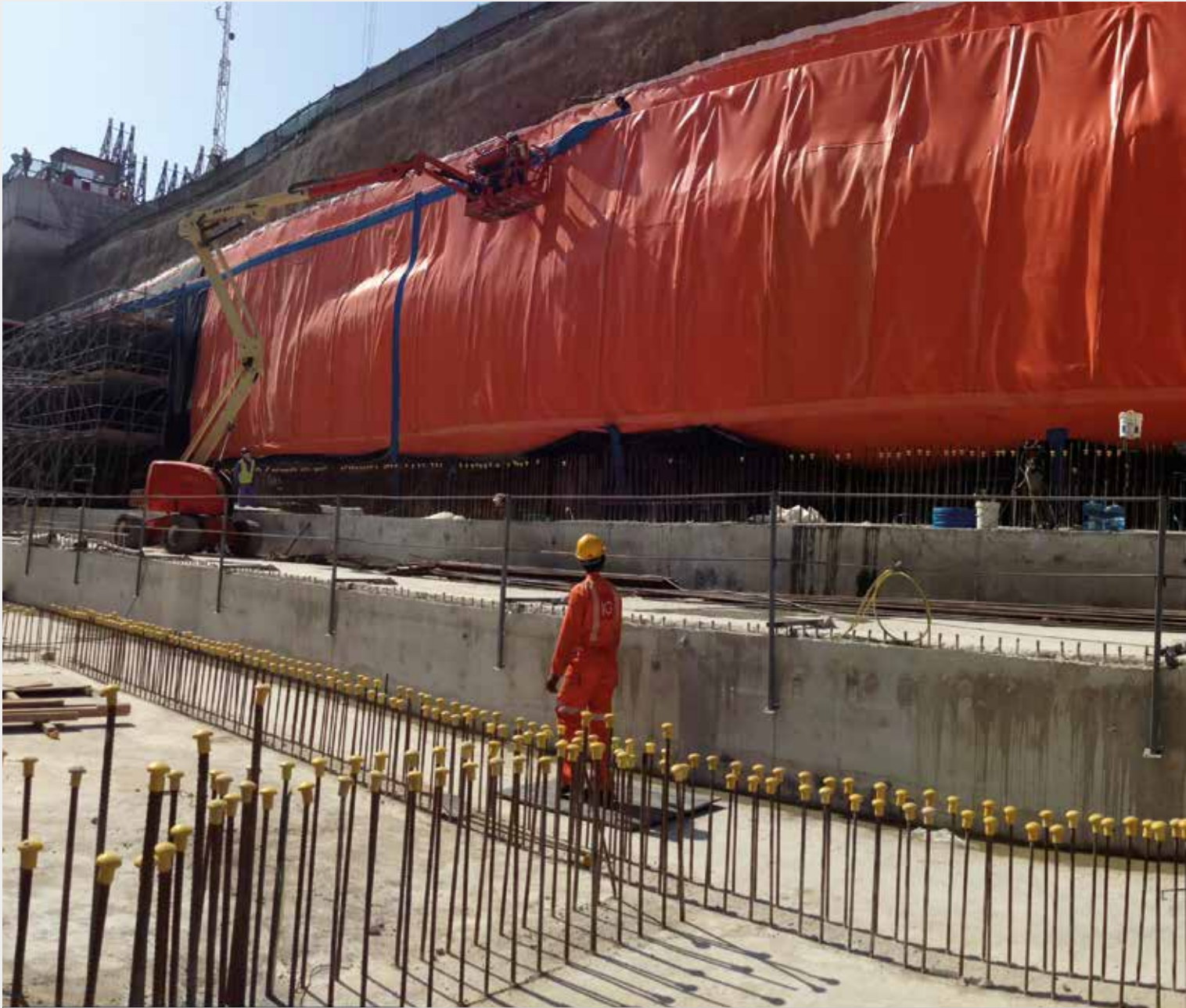
RED LINE METRO STATION - Doha - Qatar
