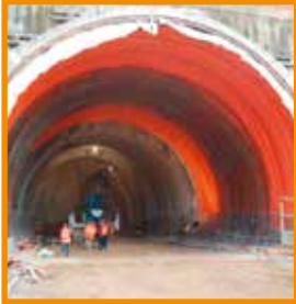
I Visual inspection
