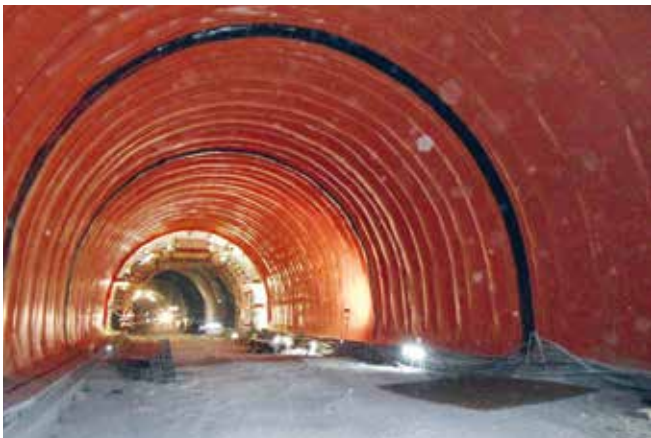
Road Tunnel (Turecky Tunnel - Slovakia)
