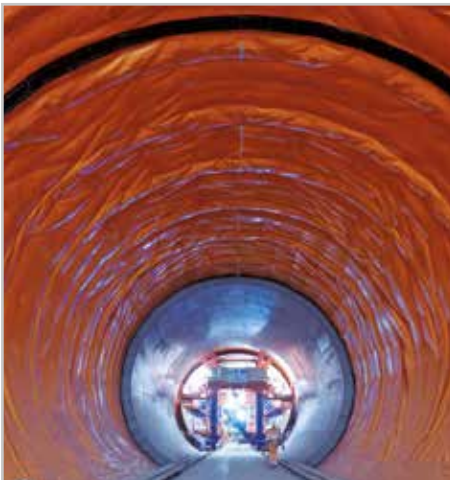
FARRINGDON STATION, Crossrail project London (UK)
