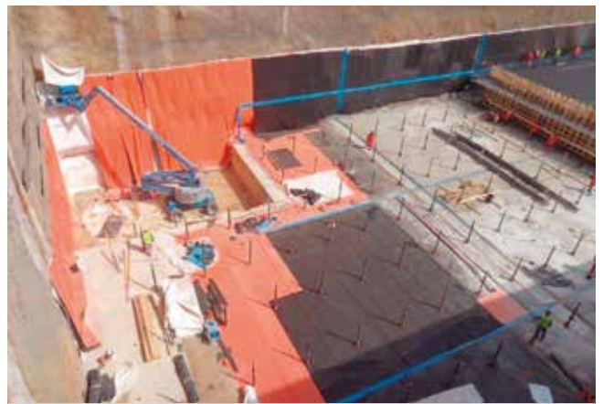
Metro Station (Riyad Metro Line 3)
