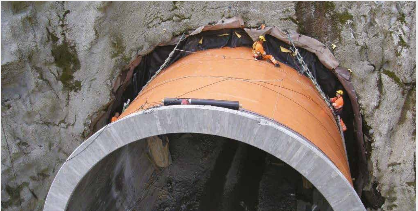
Hauge Tunnel - Istak Lonevag - Norway
