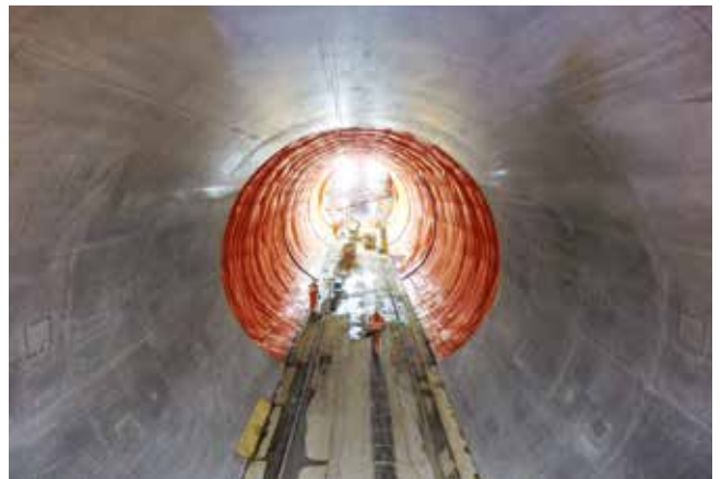
Metro Tunnel (Farringdon station - Crossrail project - London (UK))
