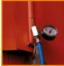
III Compressed air test – double welding
