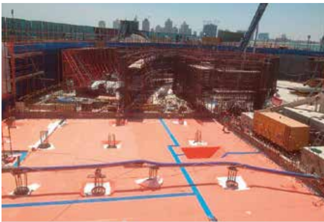
Foundation (Pearl Maison - Doha - Qatar)
