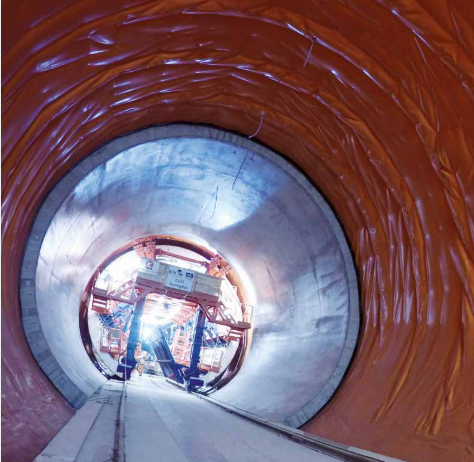
CROSSRAIL PROJECT - Farringdon Station - London (UK)
