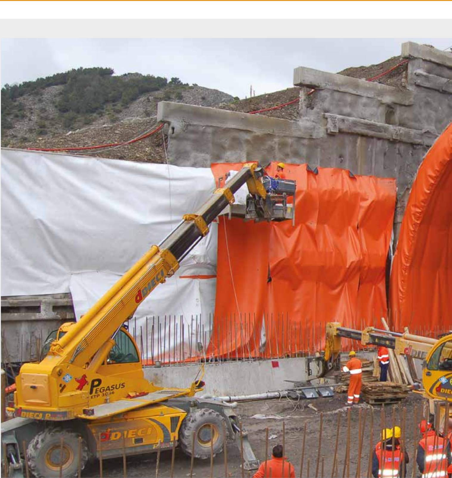
LAGONEGRO TUNNEL - Highway A3 Salerno-Reggio Calabria - Italy
