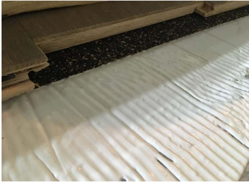
Figure 3: Mapesonic underlay adhered with Mapel Ultrabond ECO 995 adhesive .
