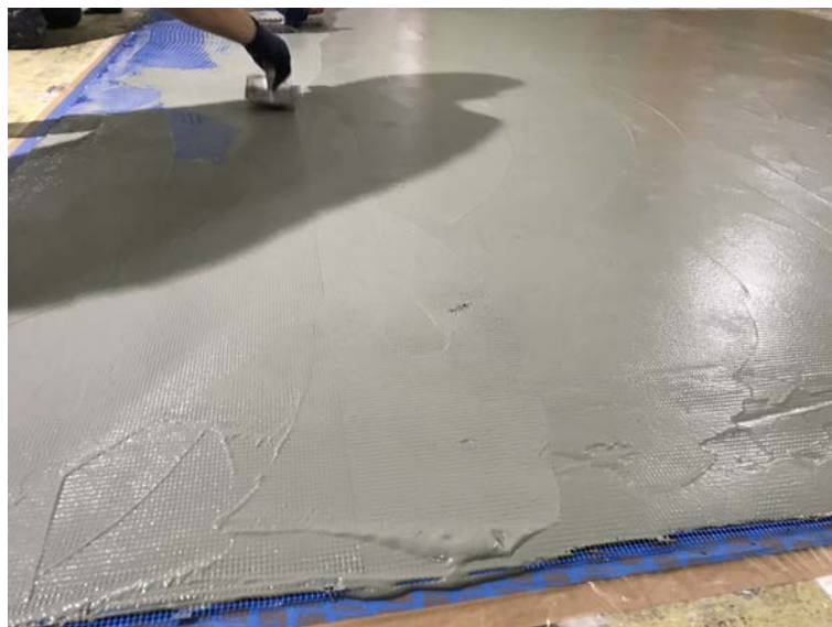
Figure 1.4: Applying Mapelastic waterproofing layer
