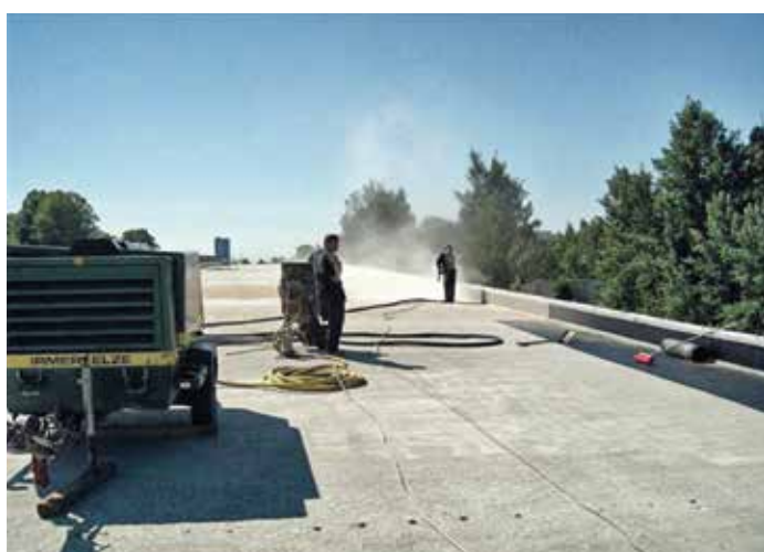
Deck cleaning with compressed air.
