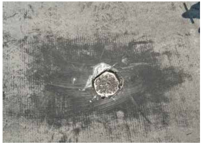
Pull-out test completed.
