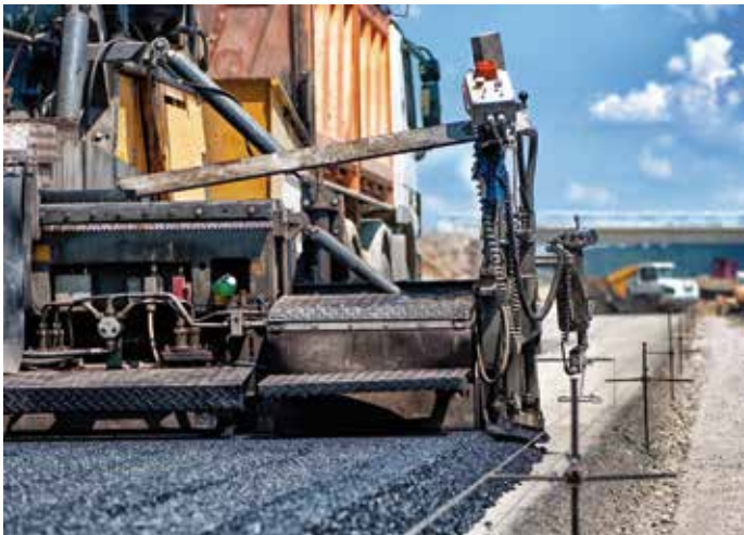
Laying of the binder course.
