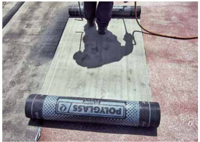
Membrane from professional line being torched on.
