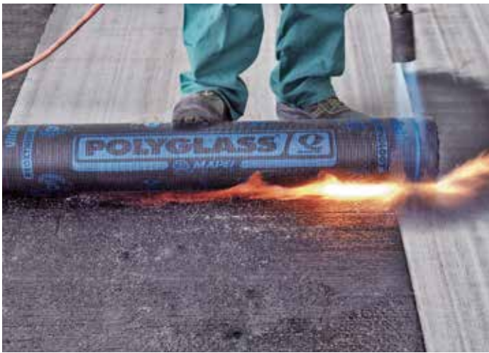
Membrane from Reoxthere line being torched on.
