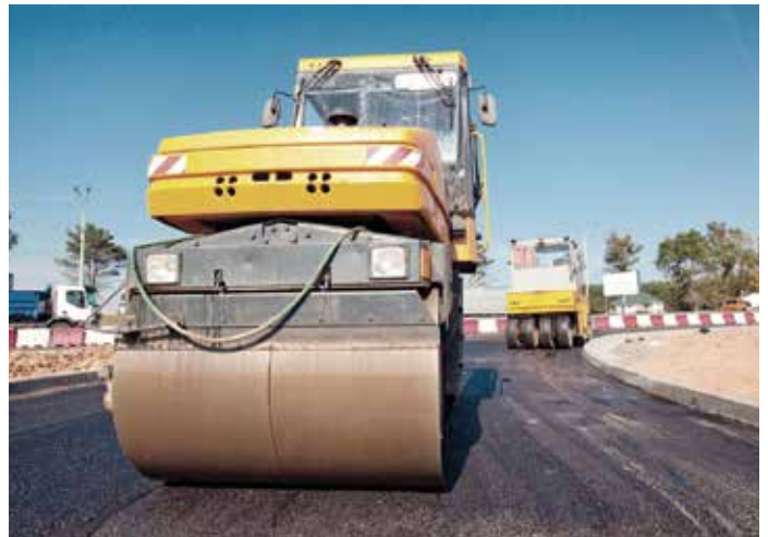
Compacting and finishing of the bituminous binder course.
