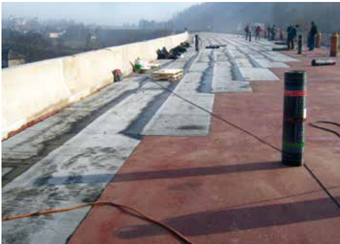
Correct staggered application of membranes.
