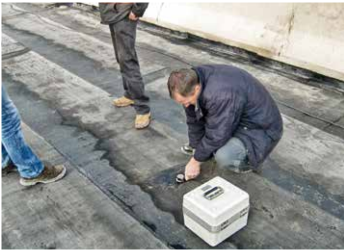
Pull-out test being performed.
