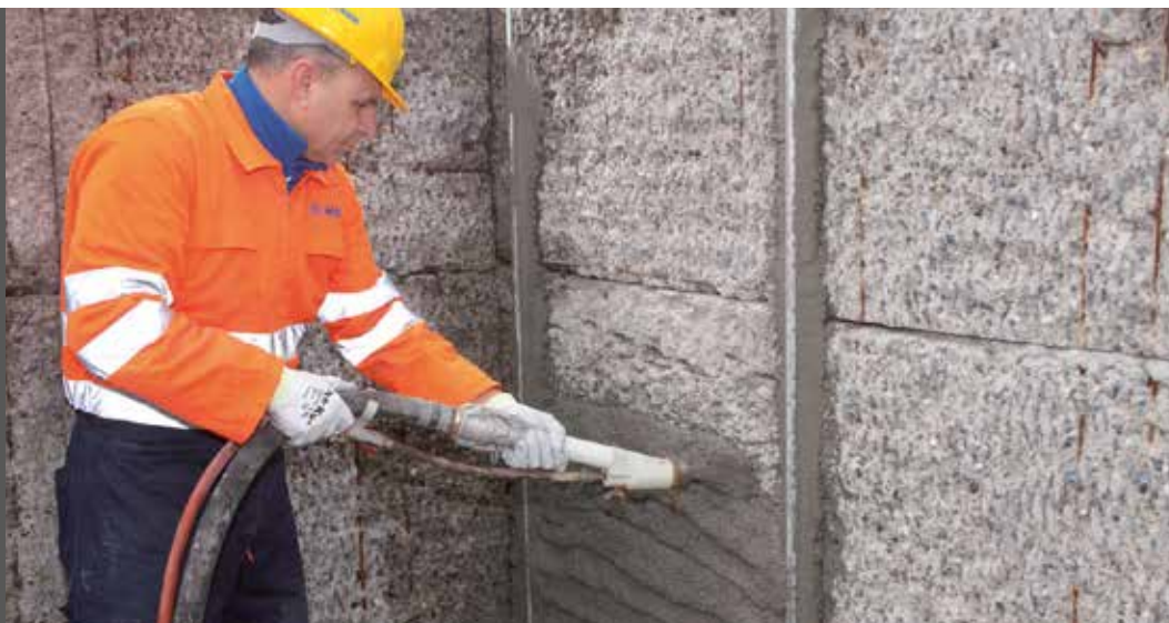
Photo 6 Application by spray of MAPEGROUT 430 , class R3 structural mortar on a concrete structure
