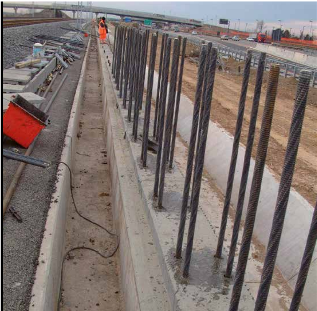
Photo 12 Anchoring steel bars in concrete using PLANIGROUT 300
