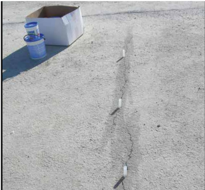
Photo 11 Injecting EPOJET in a cracked concrete slab
