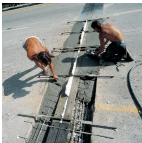
Repairing rigid joints of a highway bridge with Mapefill
