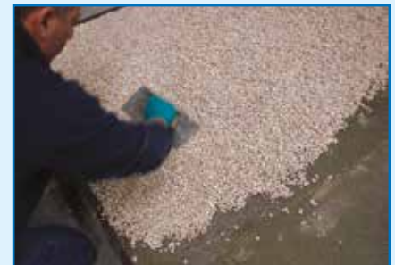
Application of the Mapefloor I 910/natural aggregates mixture
