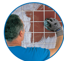
Final cleaning with a cloth
