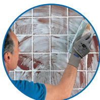
Spreading with a rubber float
