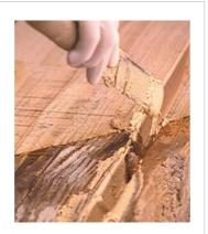
APPLICATION metal trowel 1.59 kg/dm³ of cavity to be filled CONSUMPTION PACKAGING 3 kg units:(comp. A = 2 kg; comp. B = 1 kg.
