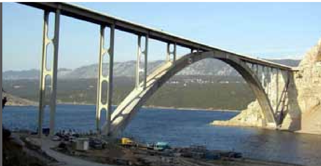
Photo 7 Large-scale concrete structure repaired with MAPEGROUT T60 , class R4 structural mortar
