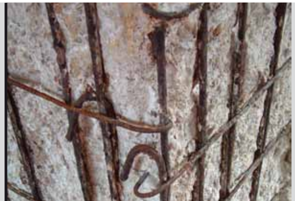
Photo 2 Example of deterioration on concrete reinforcement due to corrosion
