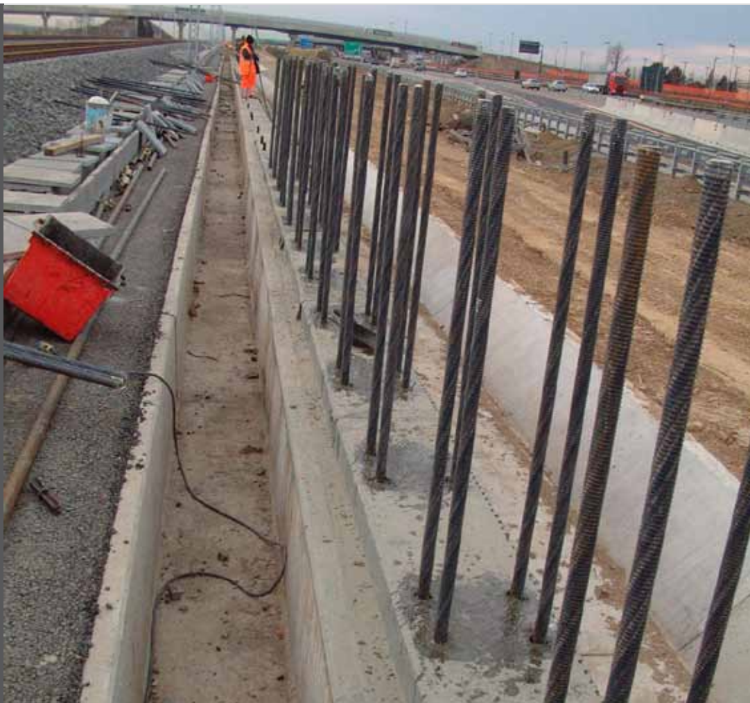
Photo 12 Anchoring steel bars in concrete using PLANIGROUT 300
