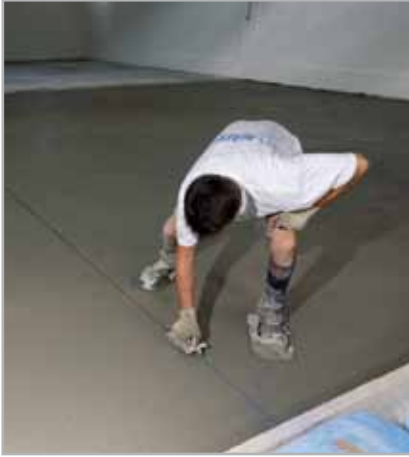
Fig. 7.8 - Forming check joints in a screed
