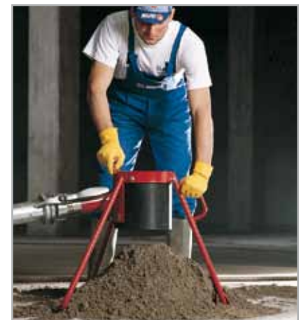
Fig. 6.2 - Batching a TOPCEM/TOPCEM PRONTO mix
