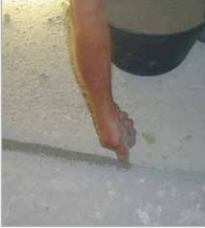
Fig. 8.4 - Sprinkling sand on the surface of fresh EPORIP
