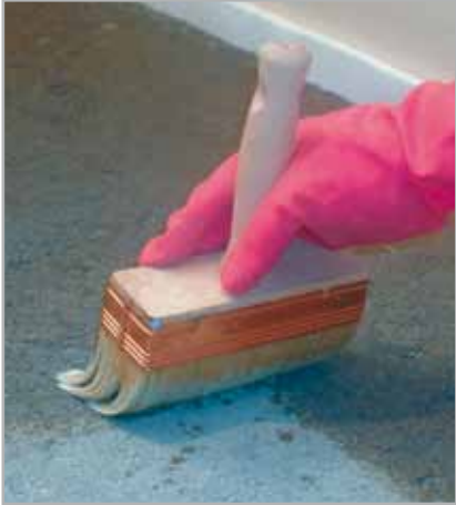
Fig. 8.13 - Brush-applying PRIMER G diluted with water on the surface of a screed
