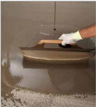
Fig. 8.14 - Creating a flat surface on a screed by applying a layer of ULTRAPLAN
