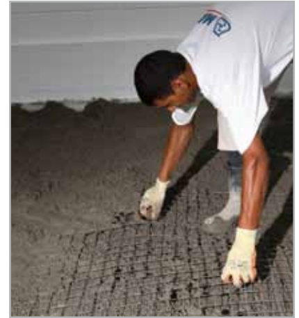
Fig. 7.5 - Placing zinc-plated metallic mesh at the mid-point of the screed
