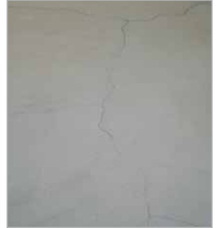
Fig. 8.1 - Cracked screed
