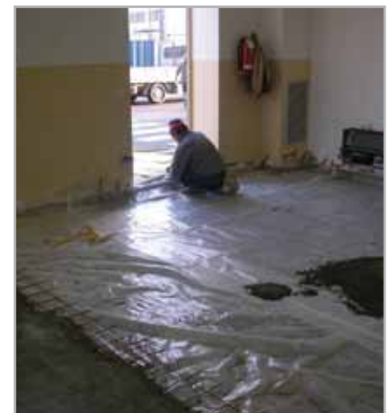
Fig. 4.2 - Laying an unbonded screed on polyethylene sheets
