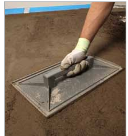
Fig. 7.6 - Float-finishing the surface of a screed
