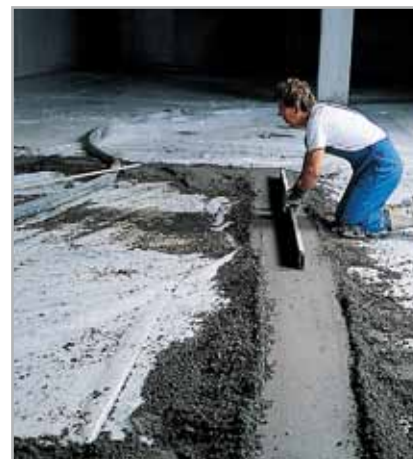
Fig. 7.1 - Forming levelling strips
