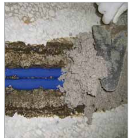
Fig. 8.8 - Filling fractures with MAPEFLOOR EP19
