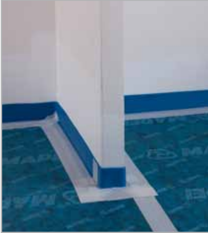
Fig. 4.9 - Floor slab isolated acoustically by laying MAPESENT ROLL, MAPESENT BAND R and MAPESENT TAPE.
