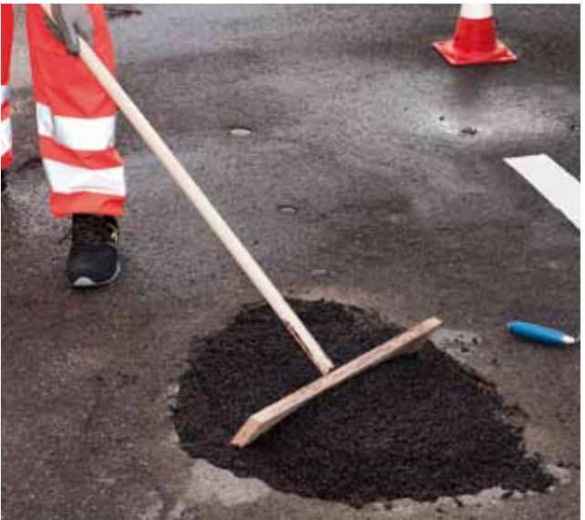
2. Applying and spreading Mape-Asphalt Repair 0/8
