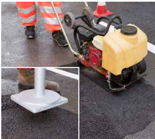
4. Manual or mechanical compacting of Mape-Asphalt Repair 0/8
