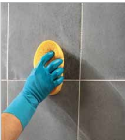
Fig. 7.25 - Finishing of the grouted joints with a sponge
