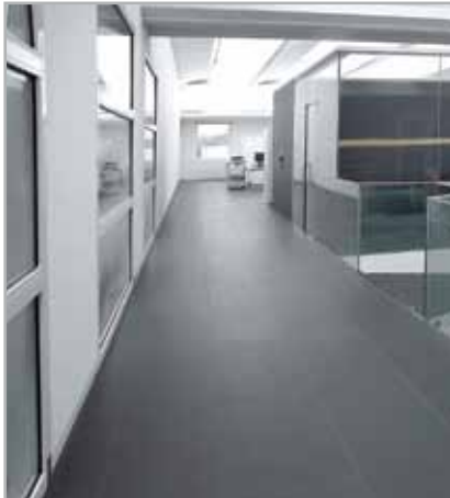
Fig. 7.8 - An example of laying thin porcelain tiles on an internal floor
