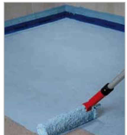
Fig. 6.2 - Application of MAPELASTIC AQUADEFENSE with a roller on a floor
