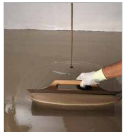
Fig. 5.2 - Levelling the surface of a cementitious screed with ULTRAPLAN
