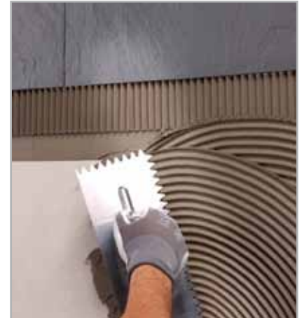
Fig. 7.4 - Fixing to walls: spreading the adhesive with a N° 6 notched trowel
