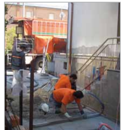
Fig. 4.4 - Mechanised system with silos mounted on a truck for storing, mixing and transporting blended TOPCEM or TOPCEM PRONTO
