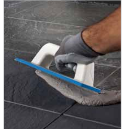
Fig. 7.20 - Grouting the joints with ULTRACOLOR PLUS
