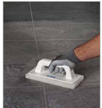
Fig. 7.21 - Cleaning with Scotch-Brite ®
