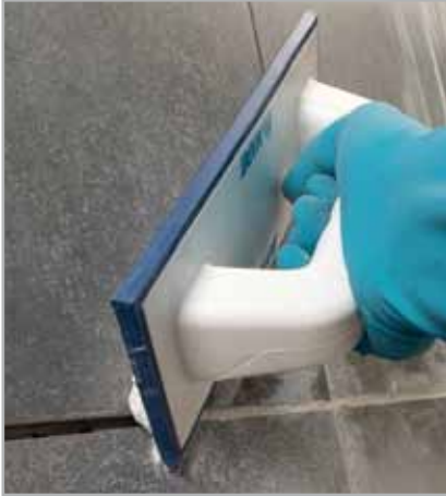
Fig. 7.23 - Grouting the tile joints on a wall with FLEXCOLOR
