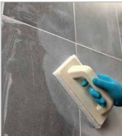
Fig. 7.24 - Cleaning with Scotch-Brite®
