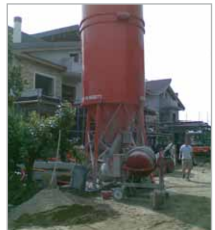
Fig. 4.3 - Mechanised system with silos for storing, mixing and transporting blended TOPCEM PRONTO
