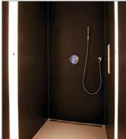
Fig. 7.15 - An example of fixing thin porcelain tiles on a waterproofing system
