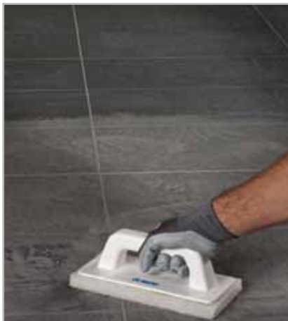
Fig. 7.19 - An example of laying thin porcelain tiles on a metal staircase
