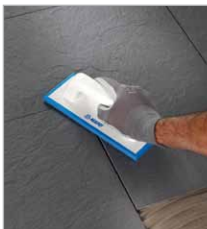
Fig. 7.3 - Laying on floors: laying and tamping the tiles in place
