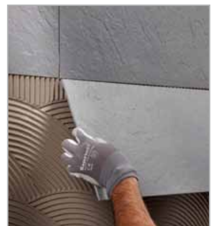
Fig. 7.6 - Fixing to walls: positioning a tile
