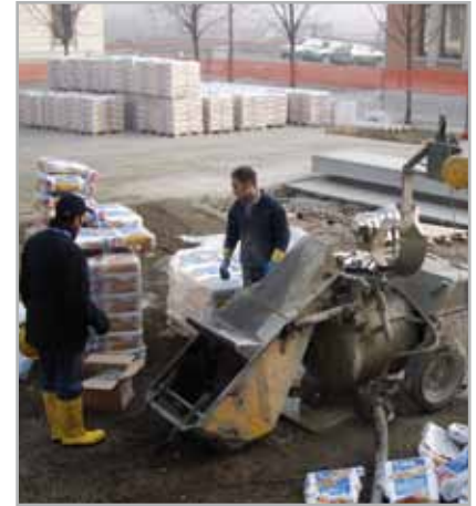
Fig. 4.2 - Mixing TOPCEM PRONTO with a pumping system
