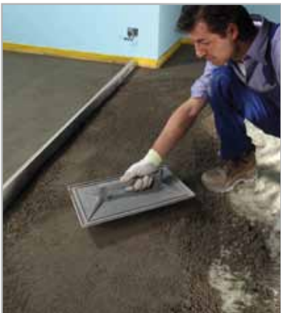
Fig. 4.6 - Tamping a screed made from TOPCEM PRONTO
