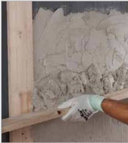
Fig. 5.5 - Evening out a concrete wall with NIVOPLAN+PLANICRETE
