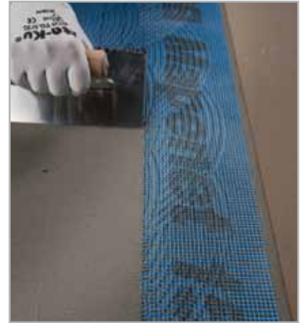
Fig. 6.1 - Application of MAPELASTIC+MAPENET 150 on a floor
