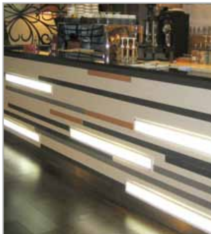
Fig. 7.18 - An example of fixing thin porcelain tiles on a wooden substrate
