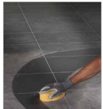
Fig. 7.22 - Finishing the grouted joints with a sponge
