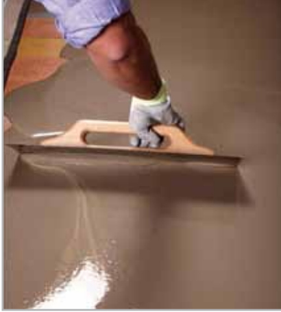
Fig. 5.4 - Levelling the surface of an old terrazzo floor with ULTRAPLAN
