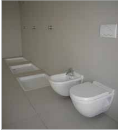
Fig. 7.14 - An example of fixing thin porcelain tiles on a waterproofing system
