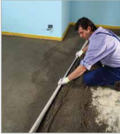
Fig. 4.5 - Levelling TOPCEM PRONTO
