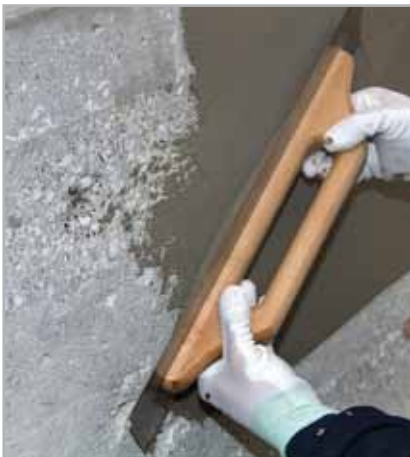
Fig. 5.6 - Evening out a wall with PLANITOP FAST 330
