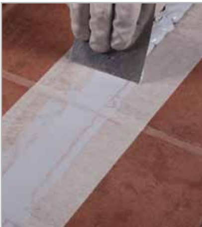
Fig. 9.6 - Smoothing over the MAPEFLEX PU40
