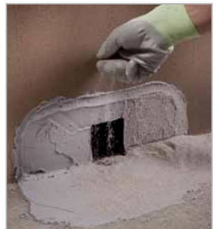
Fig. 7.6 - Sprinkling quartz on fresh ADESILEX PG4
