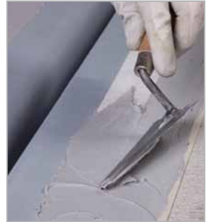
Fig. 5.16 - Applying the second layer of ADESILEX PG4
