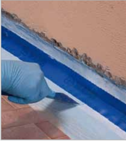
Fig. 5.25 - Embedding the white fabric of MAPEBAND in fresh MAPELASTIC AQUADEFENSE
