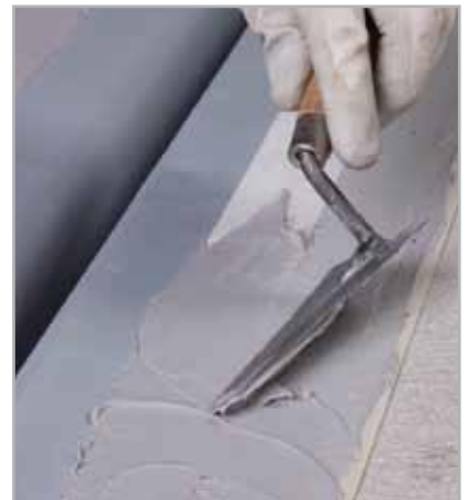
Fig. 7.11 - After laying MAPEBAND TPE on fresh ADESILEX PG4 apply the second layer
