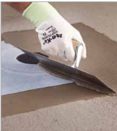
Fig. 5.62 - Application of MAPELASTIC or MAPELASTIC SMART on DRAIN VERTICAL fabric
