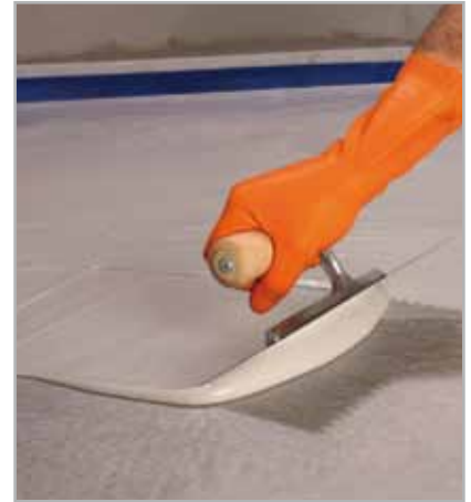
Fig. 4.13 - Second layer of MONOLASTIC applied by trowel on MAPETEX SEL
