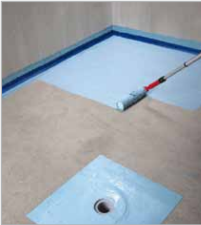
Fig. 5.56 - Application with a roller of the first coat of MAPELASTIC AQUADEFENSE
