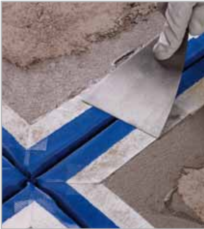
Fig. 5.68 - Embedding the white fabric of MAPEBAND in fresh MAPELASTIC or MAPELASTIC SMART
