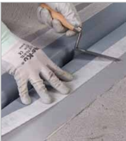
Fig. 5.15 - Applying MAPEBAND TPE on fresh ADESILEX PG4
