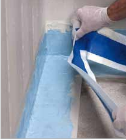
Fig. 5.55 - Application of MAPEBAND on fresh MAPELASTIC AQUADEFENSE
