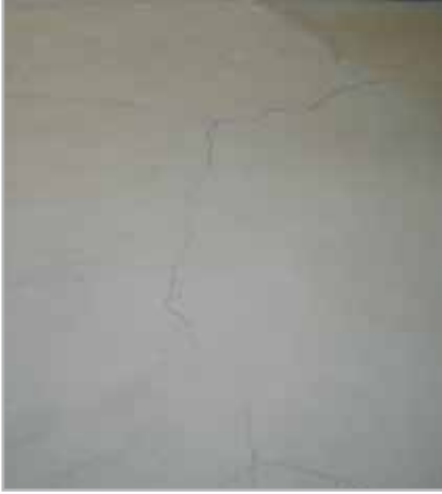
Fig. 5.1 - Cracked screed
