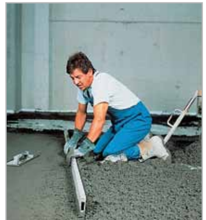
Fig. 3.8 - Levelling the surface of a TOPCEM PRONTO screed with a straight-edge
