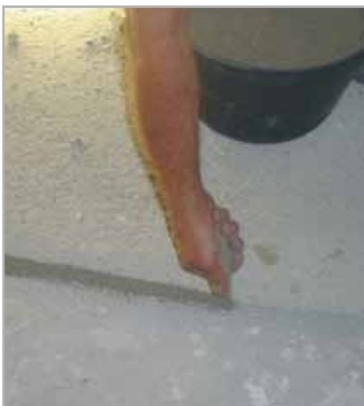
Fig. 5.33 - Sprinkling quartz on fresh EPORIP
