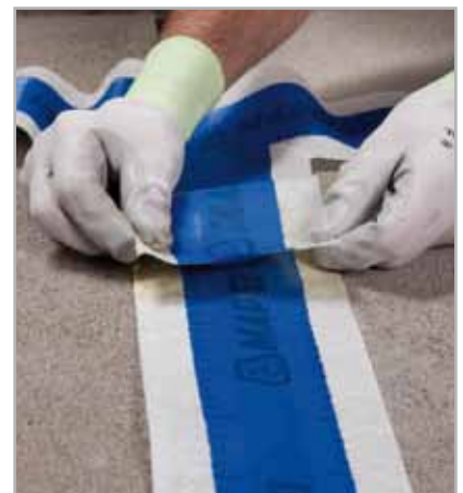
Fig. 5.42 - Bonding MAPEBAND T and MAPEBAND together by overlapping their ends
