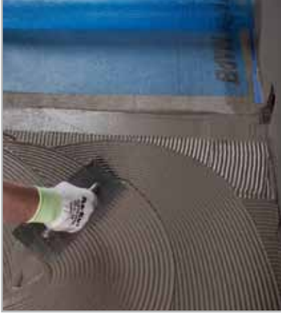
Fig. 5.49 - Application of the first coat of MAPELASTIC
