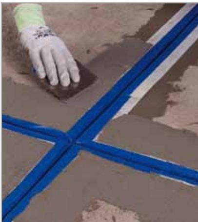
Fig. 5.69 - Application of MAPELASTIC or MAPELASTIC SMART on white MAPEBAND fabric
