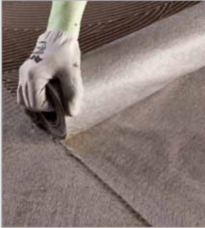
5.73 - Laying MAPETEX SEL on fresh MAPELASTIC SMART
