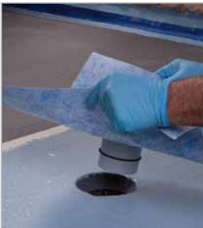
Fig. 4.17 - Application of DRAIN VERTICAL on fresh MAPELASTIC AQUADEFENSE
