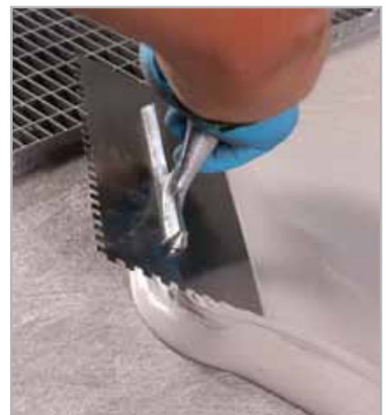
Fig. 5.23 - Second layer of MONOLASTIC applied by trowel on MAPETEX SEL
