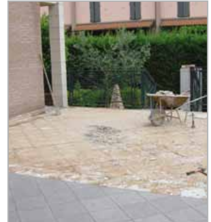
Fig. 5.28 - Removing the existing floor not bonded to the substrate
