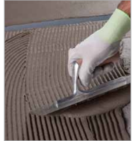
Fig. 5.46 - Spreading the first coat of MAPELASTIC starting from the structural joint
