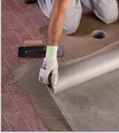
Fig. 5.19 - Applying MAPETEX SEL on fresh
