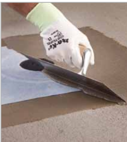
Fig. 7.3 - Application of MAPELASTIC or MAPELASTIC SMART on DRAIN VERTICAL fabric
