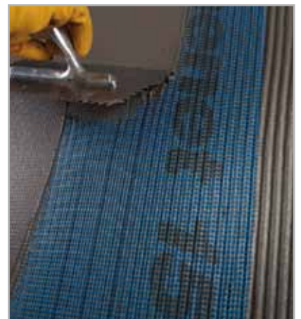
Fig. 6.9 - Embedding MAPENET 150 in the first fresh layer of MAPELASTIC
