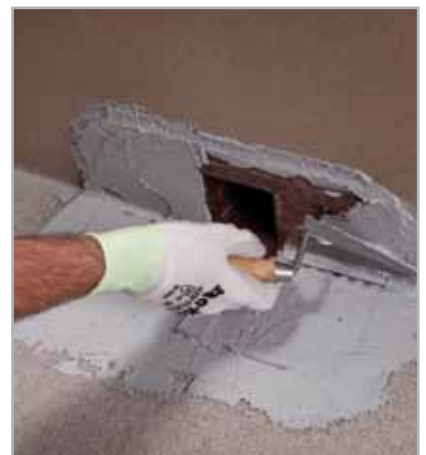
Fig. 5.65 - Application of ADESILEX PG4 to completely cover DRAIN FRONT
