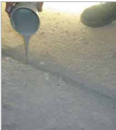
Fig. 5.32 - Sealing the cracks with EPORIP
