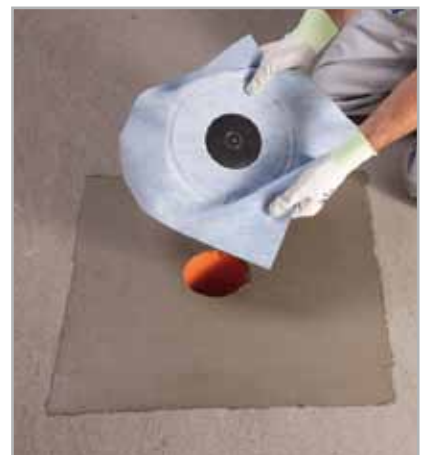
Fig. 5.59 - Positioning DRAIN VERTICAL
