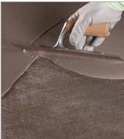
5.75 - Application of the second coat of MAPELASTIC SMART
