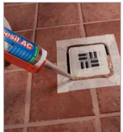
Fig. 9.2 - Sealing with MAPESIL AC
