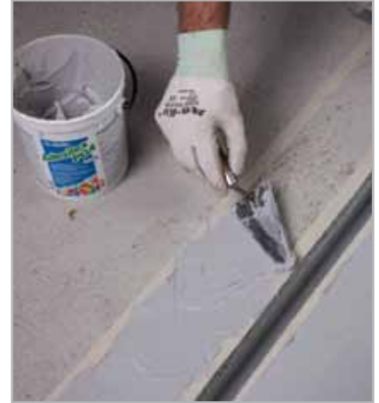
Fig. 7.10 -Applying the first layer of ADESILEX PG4
