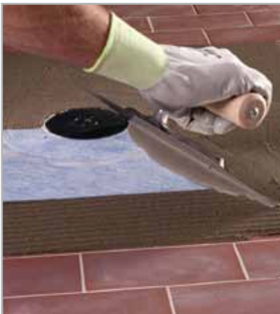
Fig. 5.9 - Applying MAPELASTIC or MAPELASTIC SMART on DRAIN VERTICAL fabric
