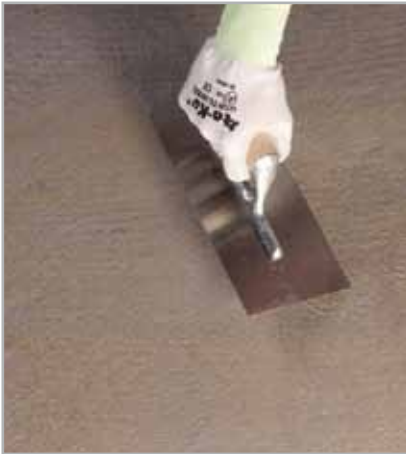
Fig. 5.20 - Embedding MAPETEX SEL in the first layer of MAPELASTIC SMART
