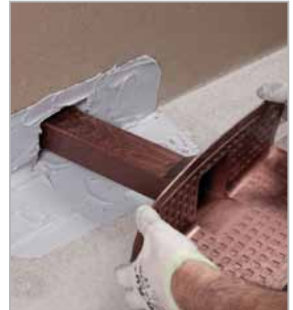
Fig. 5.10 - Application of DRAIN FRONT on fresh ADESILEX PG4
