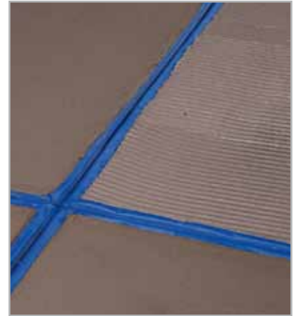
5.70 - Spreading the first coat of MAPELASTIC starting from the control joint
