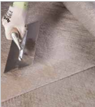
5.74 - Embedding MAPETEX SEL in the first fresh layer of MAPELASTIC SMART
