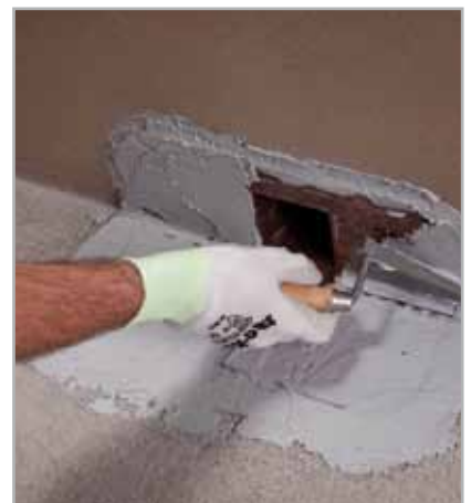
Fig. 7.5 - Application of ADESILEX PG4 to completely cover DRAIN FRONT
