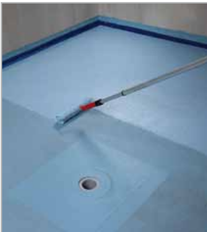
7.21 - Application with a roller of the second coat of MAPELASTIC AQUADEFENSE
