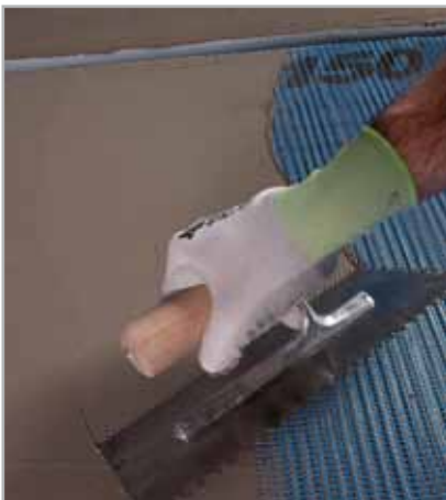
Fig. 7.14 - Embedding MAPENET 150 in the first fresh layer of MAPELASTIC
