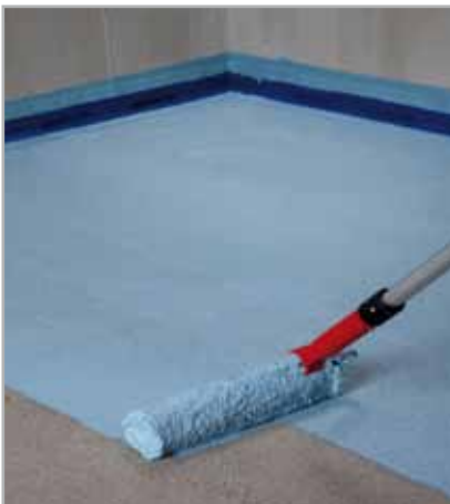
7.20 - Application with a roller of the first coat of MAPELASTIC AQUADEFENSE
