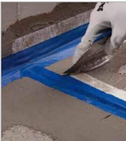
Fig. 7.8 - After embedding the white fabric of MAPEBAND T (special T-shaped piece) in the fresh product, apply MAPELASTIC or MAPELASTIC SMART on the white fabric part of MAPEBAND
