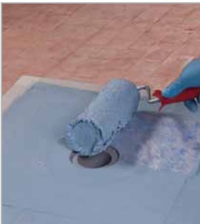
Fig. 5.26 - Complete covering of the non-woven DRAIN VERTICAL fabric with MAPELASTIC AQUADEFENSE
