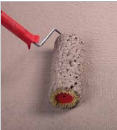
Fig. 5.51 - Application of the second layer of MAPELASTIC SMART
