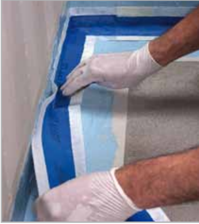
7.19 - Application of MAPEBAND on fresh MAPELASTIC AQUADEFENSE
