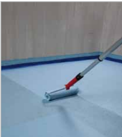
Fig. 5.57 - Application with a roller of the second coat of MAPELASTIC AQUADEFENSE
