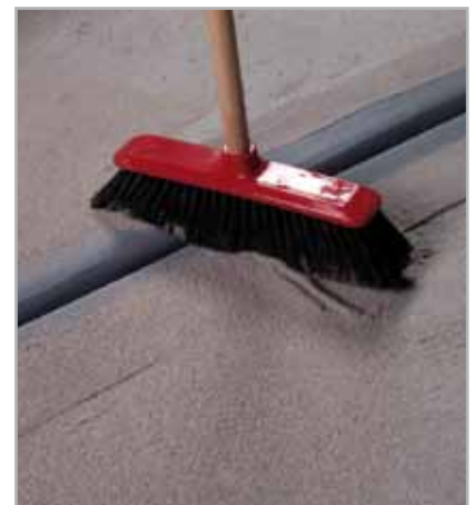
Fig. 5.18 - Removing the quartz not bonded after complete cure of ADESILEX PG4
