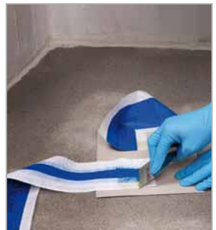
Fig. 5.54 - Spreading ADESILEX LP on the ends of MAPEBAND and MAPEBAND 90° ANGLE
