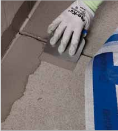
Fig. 7.7 - Application of MAPELASTIC or MAPELASTIC SMART around a control joint and a wall-floor fillet joint
