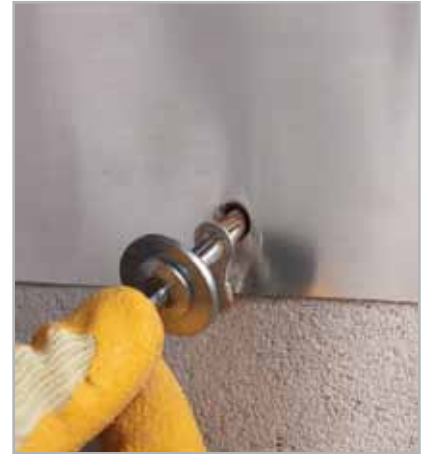
Fig. 6.7 - Fastening the metallic connectors of MAPESHIELD E 25 in place with clips
