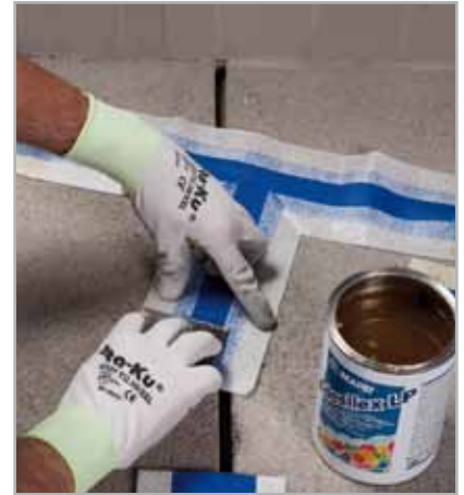
Fig. 5.40 - Spreading ADESILEX LP on MAPEBAND T
