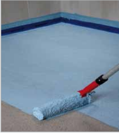
Fig. 4.4 - Application of the first coat of MAPELASTIC AQUADEFENSE
