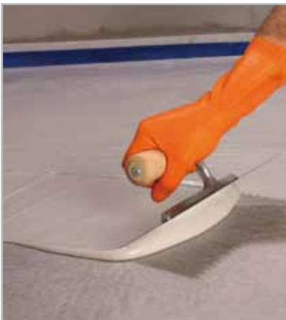
Fig. 4.5 - MONOLASTIC applied by trowel on a screed
