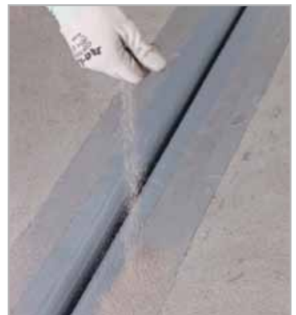
Fig. 7.12 - Sprinkling quartz on the second fresh layer
