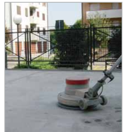
Fig. 5.29 - Sanding the substrate to remove the old adhesive from the screed
