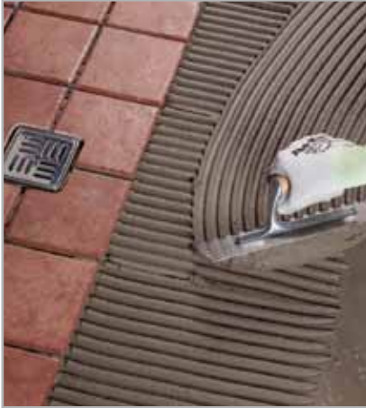
Fig. 8.4 - Bonding the tiles on perfectly dry MAPELASTIC or MAPELASTIC SMART with a class C2 adhesive
