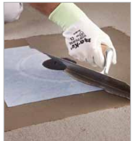
Fig. 5.36 - Applying MAPELASTIC or MAPELASTIC SMART on DRAIN VERTICAL fabric
