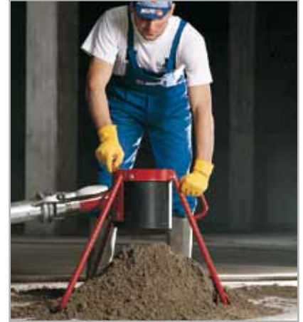
Fig. 3.7 - Applying TOPCEM PRONTO with a special pump
