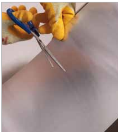
Fig. 6.4 - Cutting a self-bonding plate of pure zinc MAPESHIELD E 25
