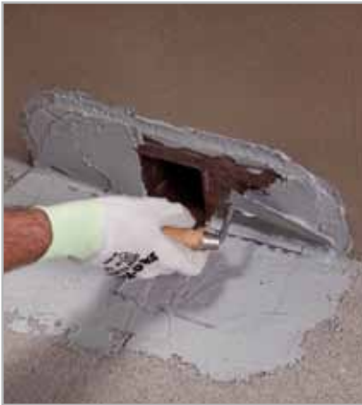
Fig. 5.38 - Application of ADÉSILEX PG4 to completely cover DRAIN FRONT
