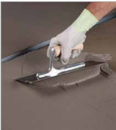
Fig. 7.15 - Application of the second coat of MAPELASTIC
