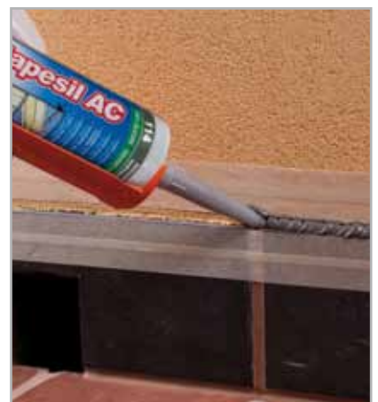
Fig. 9.3 - Sealing with MAPESIL AC
