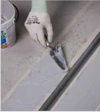
Fig. 5.43 - Applying the first layer of ADESILEX PG4
