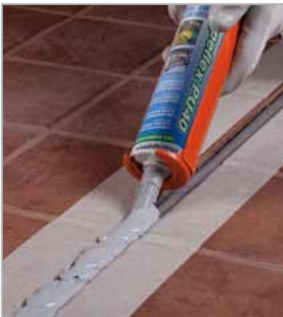
Fig. 9.5 - Sealing the structural joint with MAPEFLEX PU40
