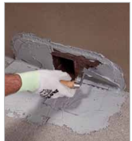
Fig. 5.11 - Application of ADESILEX PG4 to completely cover DRAIN FRONT
