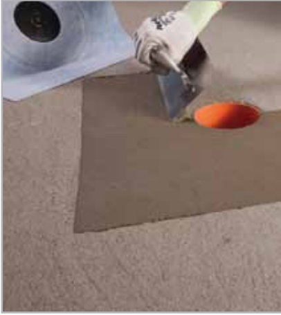
Fig. 7.1 - Applying MAPELASTIC or MAPELASTIC SMART around a floor drain
