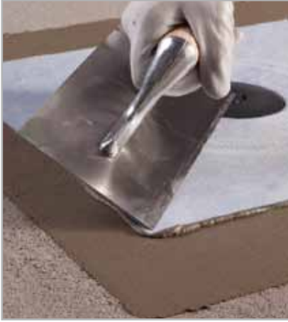
Fig. 5.61 - Press the non-woven DRAIN VERTICAL fabric on MAPELASTIC or MAPELASTIC SMART
