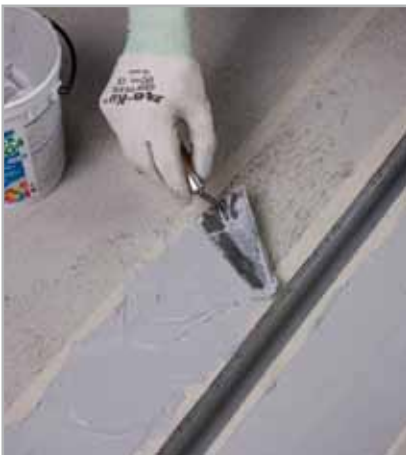
Fig. 5.14 - Applying the first layer of ADESILEX PG4
