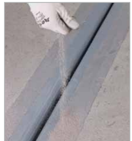
Fig. 5.17 - Sprinkling quartz on the second fresh layer
