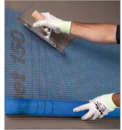
Fig. 4.1 - Application of MAPELASTIC reinforced with MAPENET 150 on a substrate with crazed cracking
