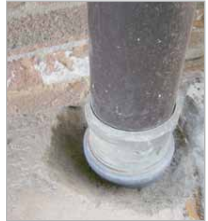
Fig. 5.4 - Demolition around a drain-pipe
