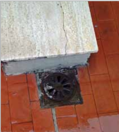
Fig. 5.2 - Floor drain with infiltrations
