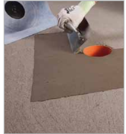
Fig. 5.58 - Applying MAPELASTIC or MAPELASTIC SMART around a floor drain
