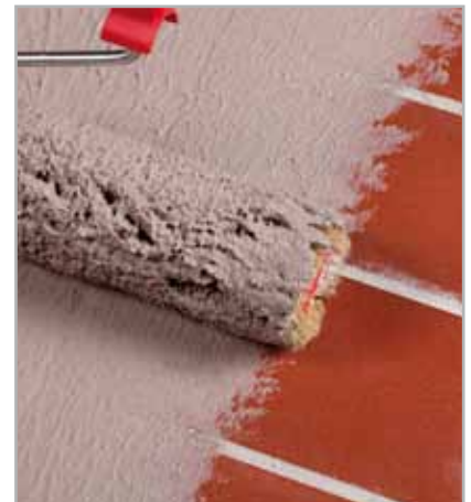
Fig. 4.2 - MAPELASTIC SMART applied with a roller on existing floor
