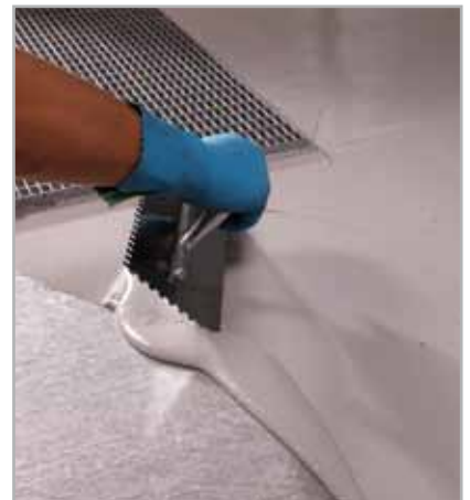
7.17 - Application of a second coat of MONOLASTIC by trowel on MAPETEX SEL
