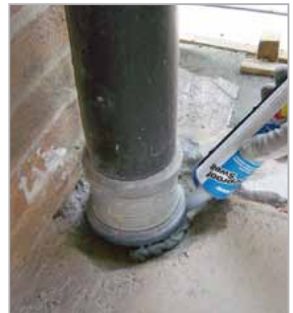
Fig. 5.5 - Extrusion of MAPEPROOF SWELL
