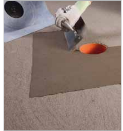
Fig. 5.34 - Applying MAPELASTIC or MAPELASTIC SMART around a floor drain
