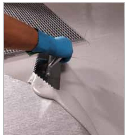
Fig. 4.14 - Second layer of MONOLASTIC applied by trowel on MAPETEX SEL
