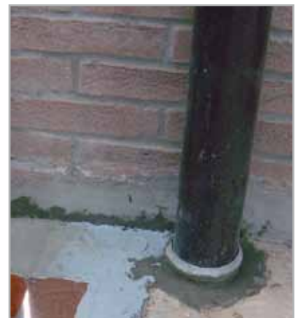
Fig. 5.6 - Repairs to a substrate using MAPEGROUT 430
