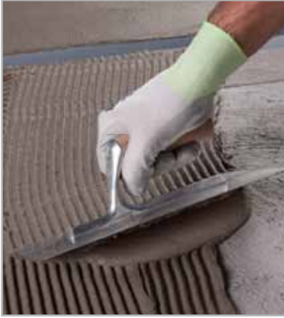
Fig. 7.13 - Spreading the first coat of MAPELASTIC starting from the structural joint
