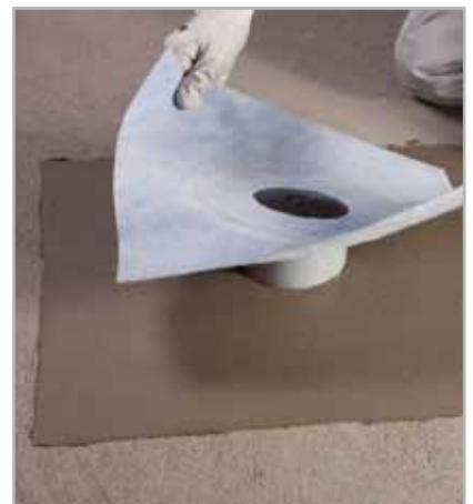
Fig. 5.60 - Inserting DRAIN VERTICAL on fresh MAPELASTIC or MAPELASTIC SMART
