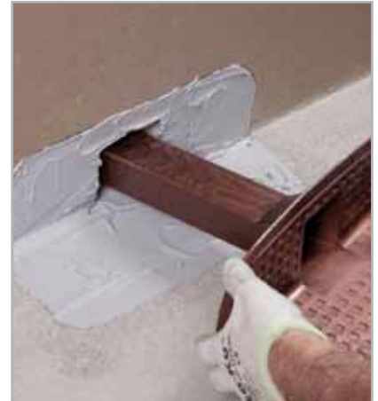
Fig. 7.4 - Application of DRAIN FRONT on fresh ADESILEX PG4
