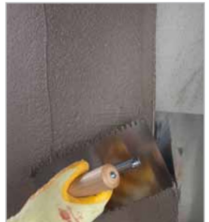
Fig. 6.8 - Protection and smoothing of the surface of MAPELASTIC
