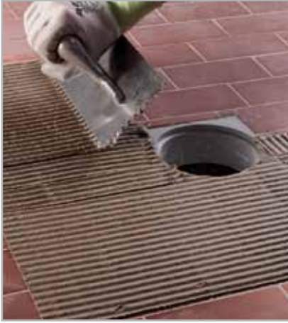
Fig. 5.7 - Applying MAPELASTIC or MAPELASTIC SMART around a floor drain
