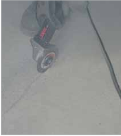
Fig. 5.31 - Opening the cracks in the screed with a grinder
