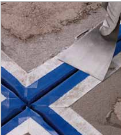
Fig. 7.9 - Embedding the white fabric of MAPEBAND CROSS (special cross-shaped piece) in fresh MAPELASTIC or MAPELASTIC SMART
