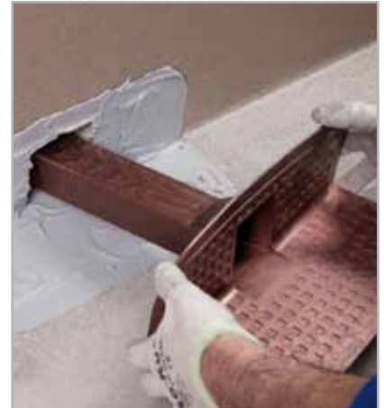
Fig. 5.64 - Application of DRAIN FRONT on fresh ADESILEX PG4
