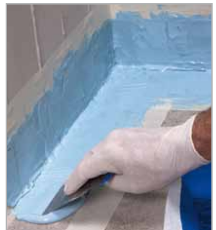
7.18 - MAPELASTIC AQUADEFENSE applied on a floor-wall fillet joint before applying MAPEBAND
