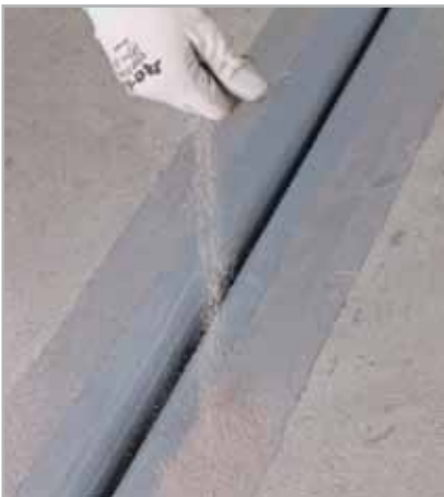
Fig. 5.45 - Sprinkling quartz on the second fresh layer
