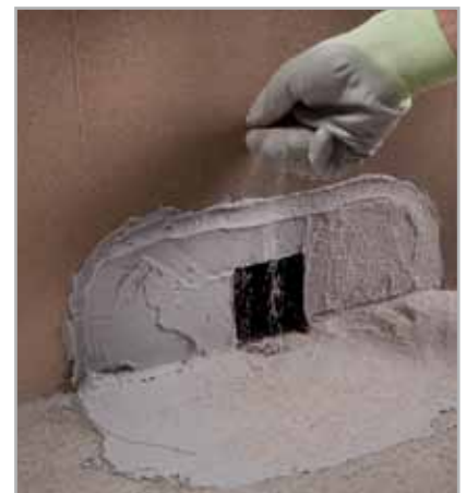
Fig. 5.12 -Sprinkling quartz on fresh ADESILEX PG4
