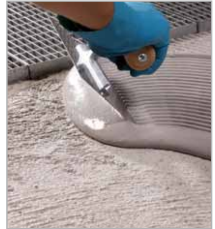
Fig. 5.22 - Second layer of MONOLASTIC applied by trowel on MAPETEX SEL
