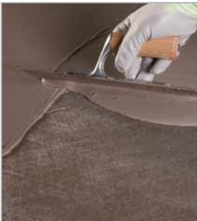
Fig. 5.21 - Applying the second layer of MAPELASTIC SMART
