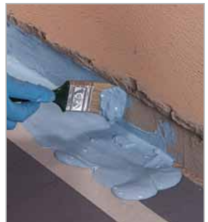
Fig. 4.15 - MAPELASTIC AQUADEFENSE applied by brush on a floor-wall fillet joint before applying MAPEBAND
