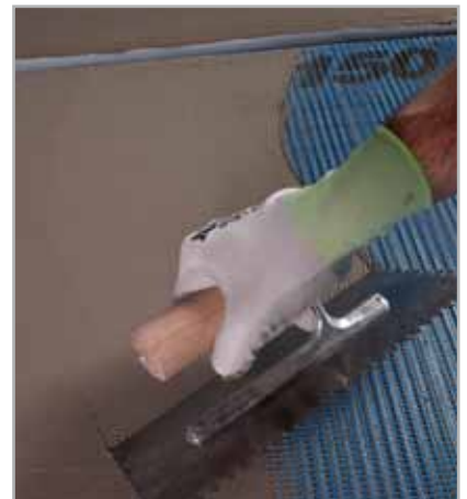
Fig. 5.47 - Impregnating MAPENET 150 in the first fresh layer of MAPELASTIC
