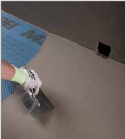
Fig. 5.50 - Embedding MAPENET 150 in the first fresh layer of MAPELASTIC
