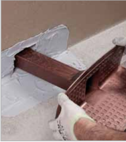
Fig. 5.37 - Application of DRAIN FRONT on fresh ADÉSILEX PG4
