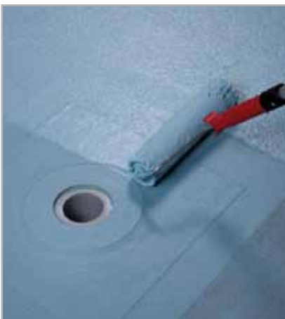
Fig. 5.27 - Application with a roller of the second coat of MAPELASTIC AQUADEFENSE
