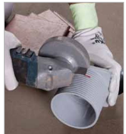
Fig. 8.2 - Cutting the telescopic extension for the grate to the length measured in the previous step
