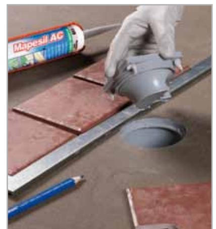
Fig. 8.3 - Bonding the telescopic extension for the grate (with anti-odour plug in place) with four spots of MAPESIL AC silicone sealant
