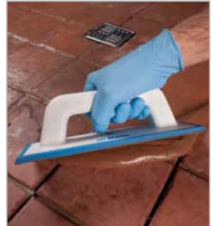
Fig. 9.1 - Grouting the joints
