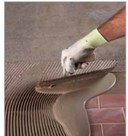
Fig. 4.3 - MAPELASTIC SMART applied with a trowel on existing floor
