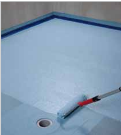
Fig. 4.18 - Application with a roller of the second coat of MAPELASTIC AQUADEFENSE
