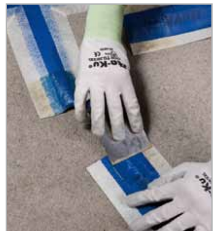
Fig. 5.41 - Spreading ADESILEX LP on MAPEBAND
