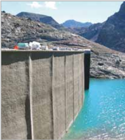
Fig. 4.11 - Example of application of MAPELASTIC: dam
