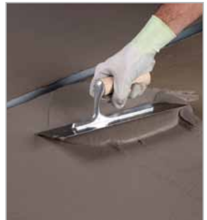
Fig. 5.48 - Application of the second coat of MAPELASTIC
