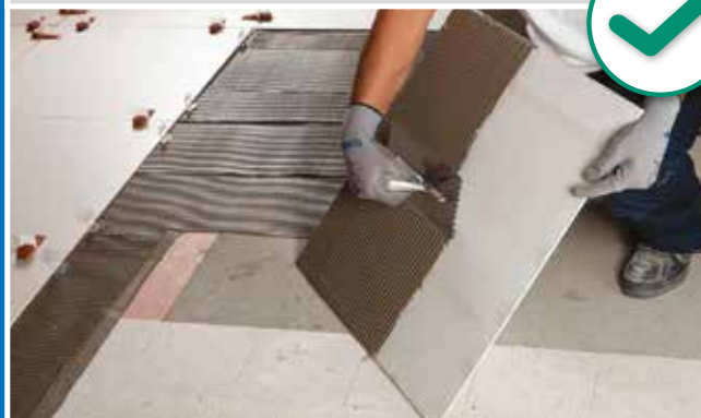
Posa conforme a UNI 11493
