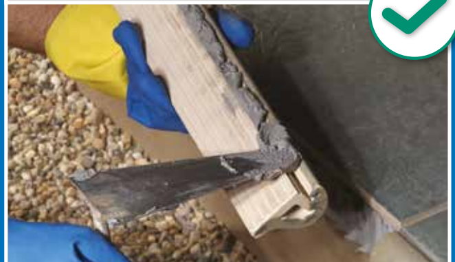
Posa conforme a UNI 11493
