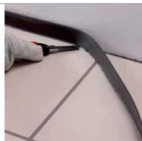
Fig. 5.8 - Grout the surface and trim the excess of MAPESONIC STRIP
