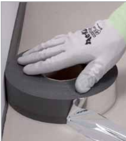
Fig. 5.2 - Apply MAPESONIC STRIP around the perimeter
