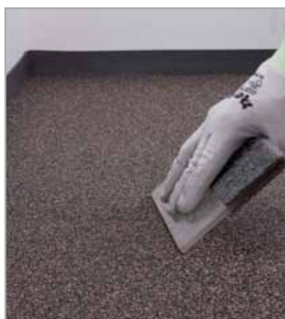
Fig. 5.5 - Massage the surface of MAPESONIC CR
