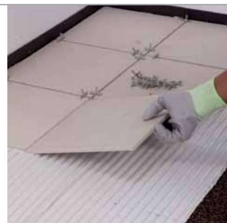
Fig. 5.6 - Spread the adhesive to bond ceramic tiles
