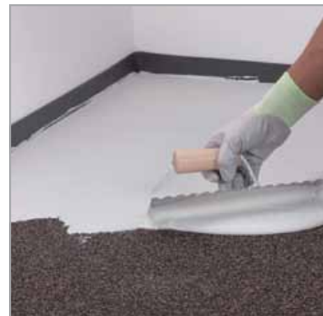
Fig. 5.4 - Unroll the sheets of MAPESONIC CR
