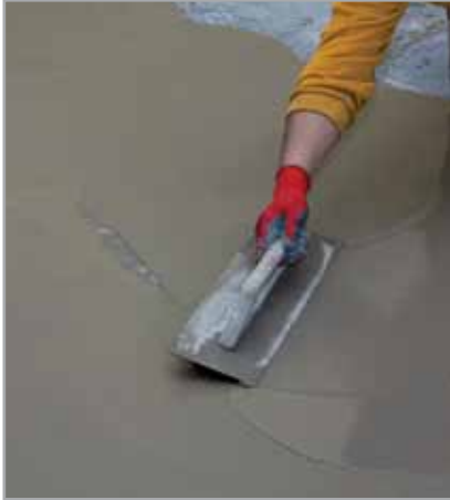
Fig. 5.1 - Levelling of the substrate
