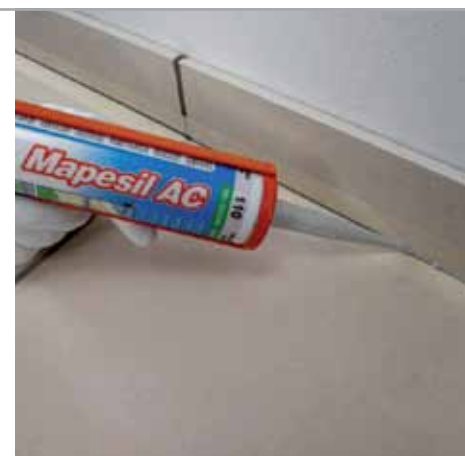
Fig. 5.9 - Apply the skirting board and seal with a suitable elastic sealant
