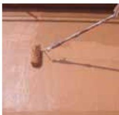
Applying the membrane
