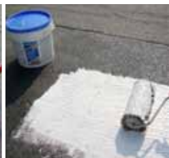
Applying the membrane
