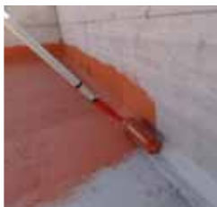
Applying the membrane
