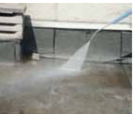
Cleaning the substrate
