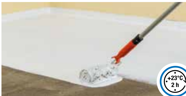
Application of the first coat
