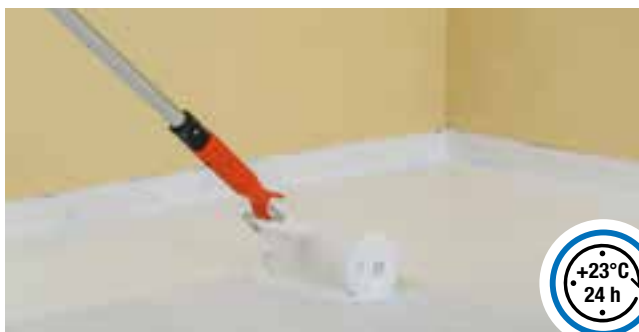
Application of the second coat
