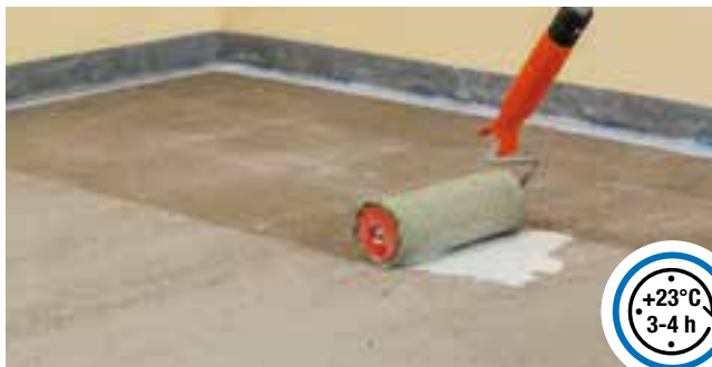
Priming the substrate
