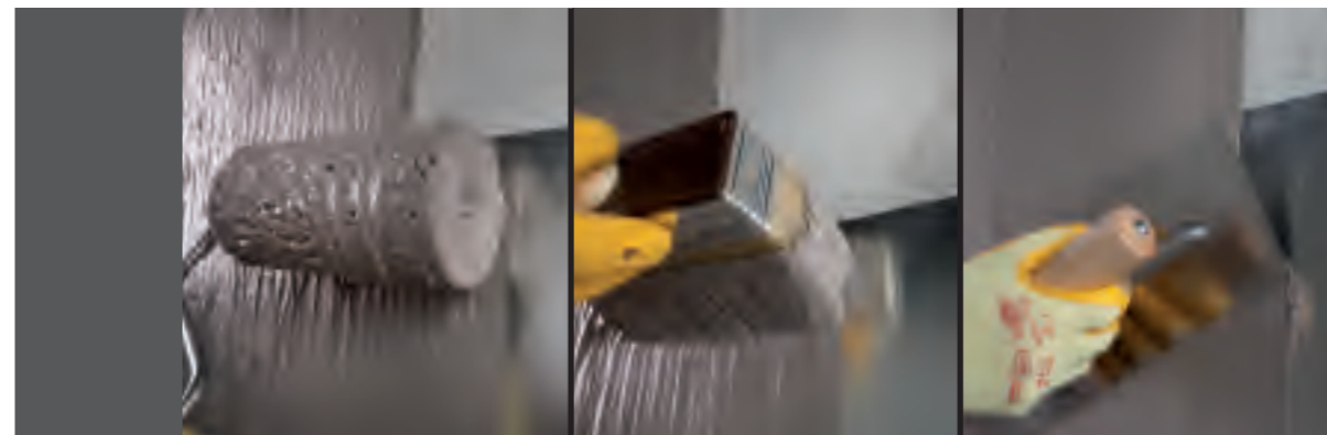
Photos 10 - 11 - 12 Smoothing over and protecting MAPESHIELD E25 :
