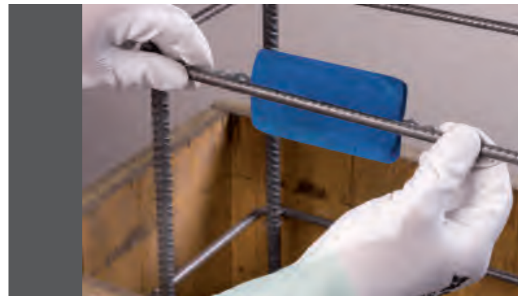
Photo 5 Application of MAPESHIELD I on a new structure
