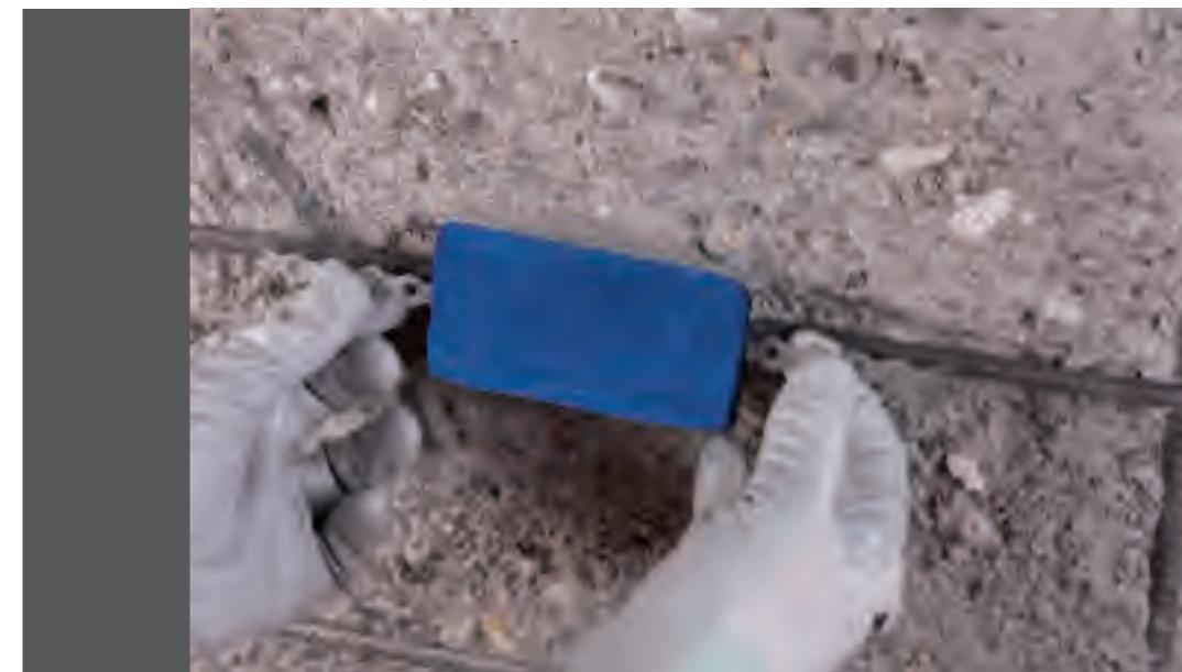
Photo 4 Application of MAPESHIELD I on a structure under repair
