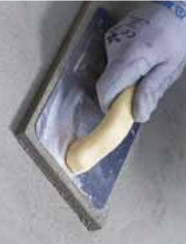
Floating the surface of Plantop Smooth & Repair R4
