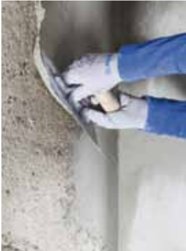
Application of Plantop Smooth & Repair R4 with a finishing trowel
