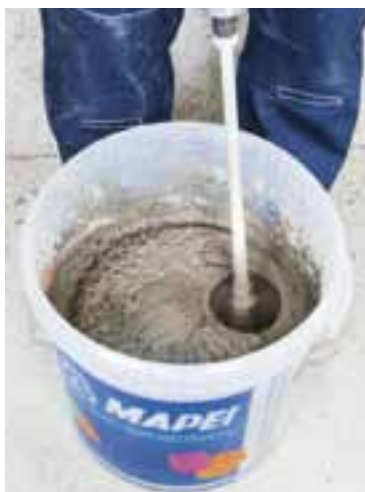
Mixing Planitop Smooth & Repair
