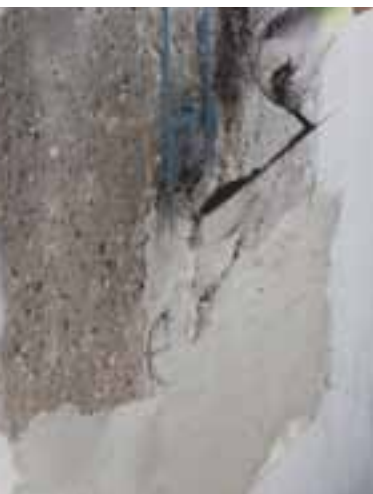
Application of Planitop Smooth & Repair by trowel
