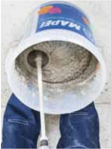
Mixing Planitop Smooth & Repair R4
