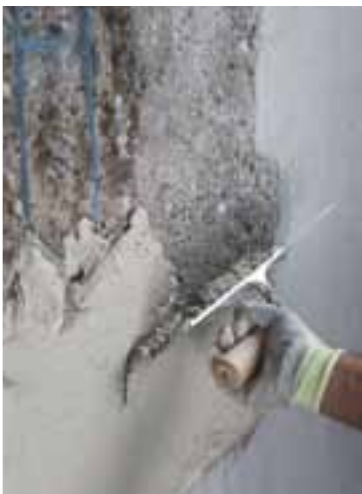
Application of Planitop Smooth & Repair with a finishing trowel
