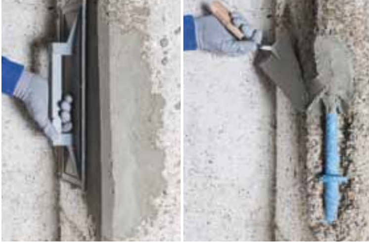
Application of Planitop Smooth & Repair R4 by trowel
