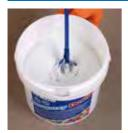
Pour all the catalyser (component B) into the container of component A and blend together with a mixer at low-speed to form a smooth paste. Never use partial quantities of the components otherwise the grout may not harden correctly. When using **Kerapoxy Design**, various amounts of **MapeGlitter** may be added according to the effect required.
