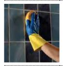
Remove any excess liquid from the surface with a hard, cellulose sponge (such as a MAPEI sponge). Replace the sponge when it is too impregnated with resin. It is important that there are no traces of grout on the surface of the tiling after the cleaning operation. Once hardened it is very difficult to remove, which is why the sponge must be rinsed frequently.
