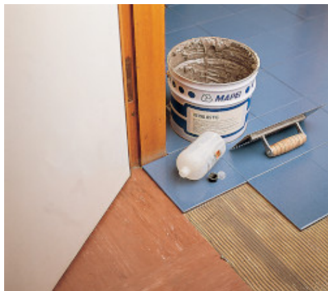
Laying on an old PVC floor
