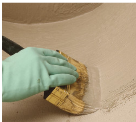
Waterproofing of details by brush
