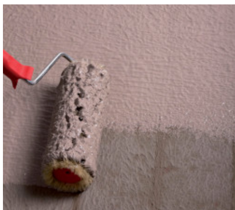
Waterproofing of terraces by roller
