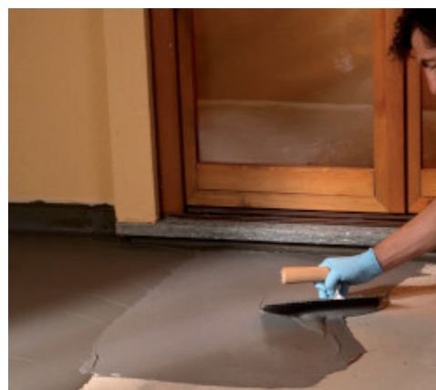
Waterproofing of terraces by trowel
