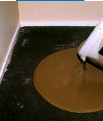
Applying the Novoplan 21CN paste on the substrate
