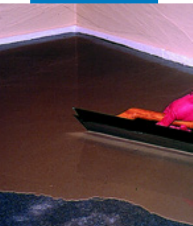
Applying Novoplan 21 CN with a metal trowel on a cementitious screed primed with Primer G
