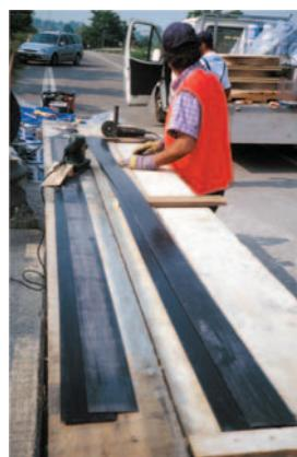
Obr. 17: Příprava lamely CARBOPLATE
