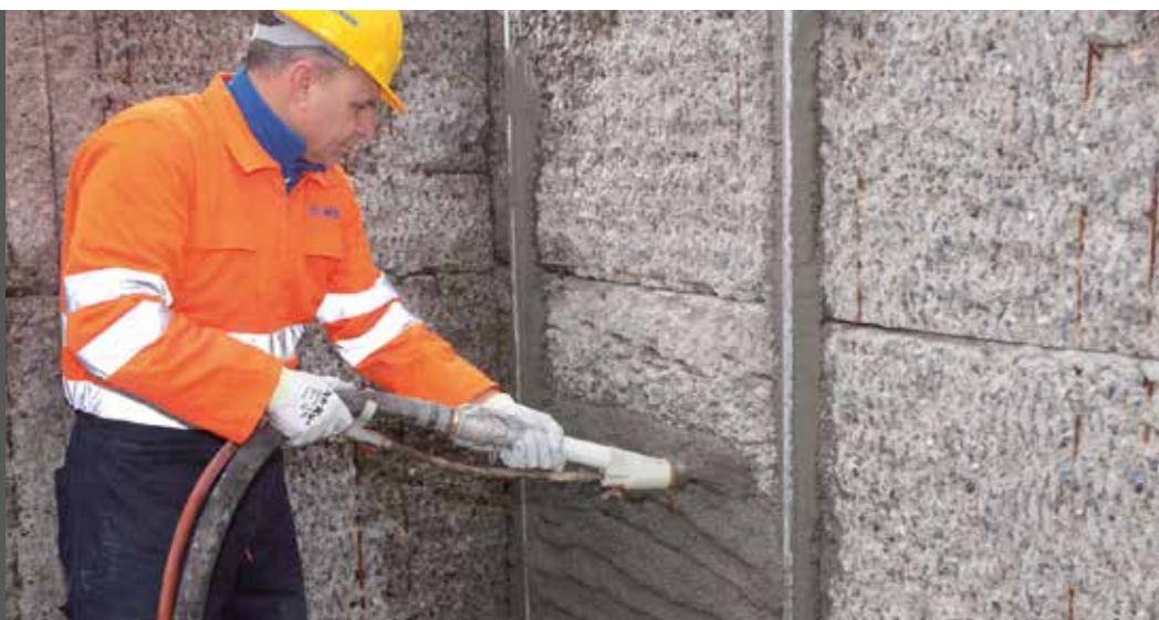
Photo 6 Application by spray of MAPEGROUT 430 , class R3 structural mortar on a concrete structure
