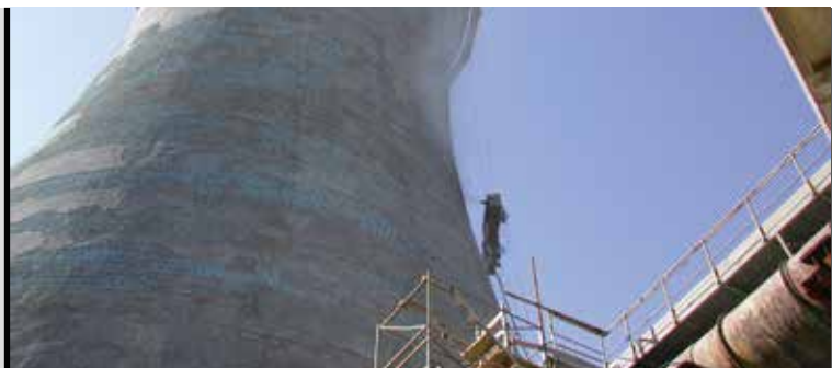
Photo 14 Reinforcement bars on a cooling tower treated with MAPEFER 1K
