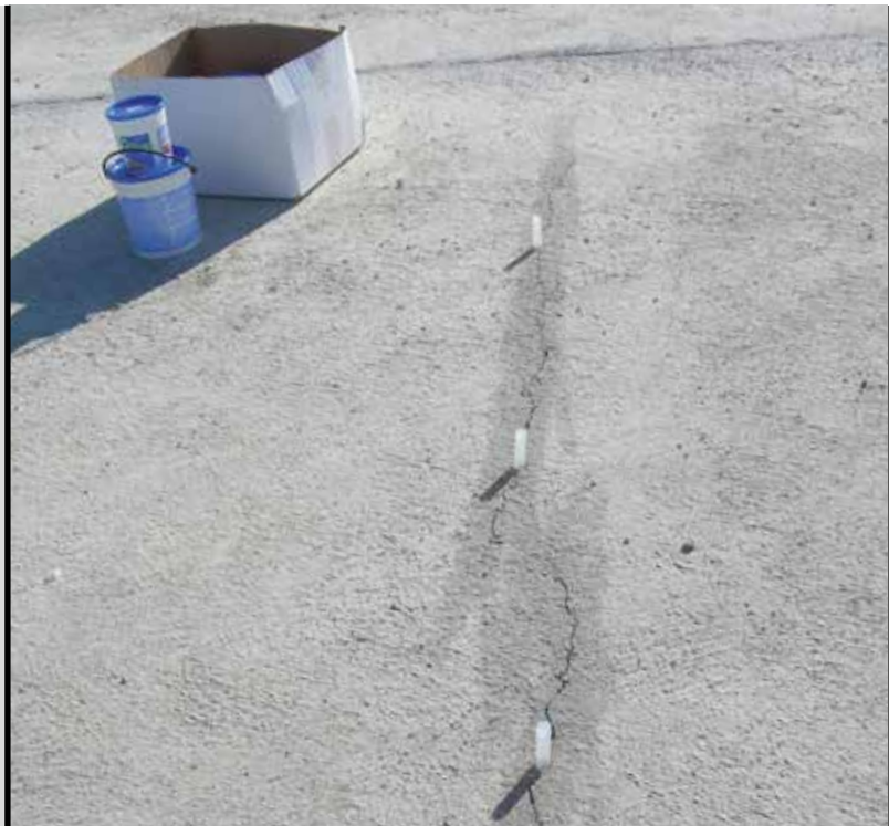
Photo 11 Injecting EPOJET in a cracked concrete slab
