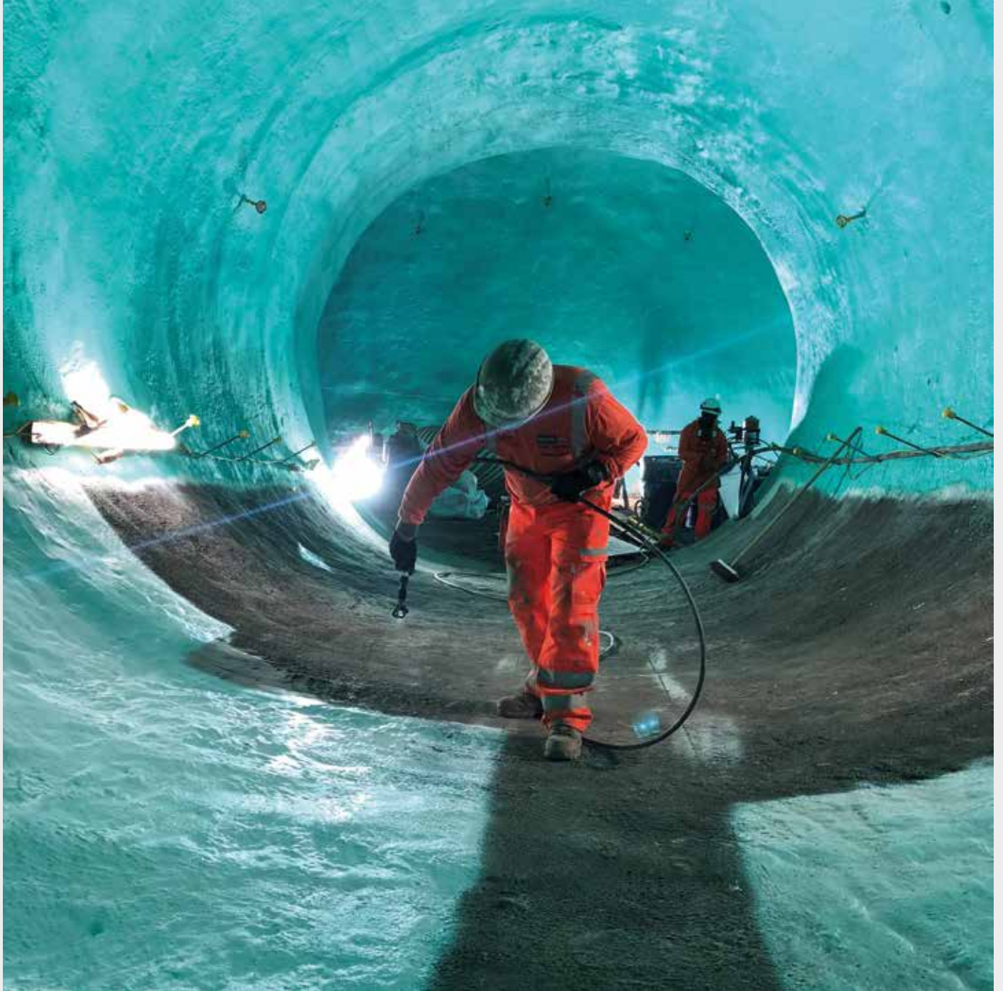
BANK STATION CAPACITY UPGRADE PROJECT, London (UK)
