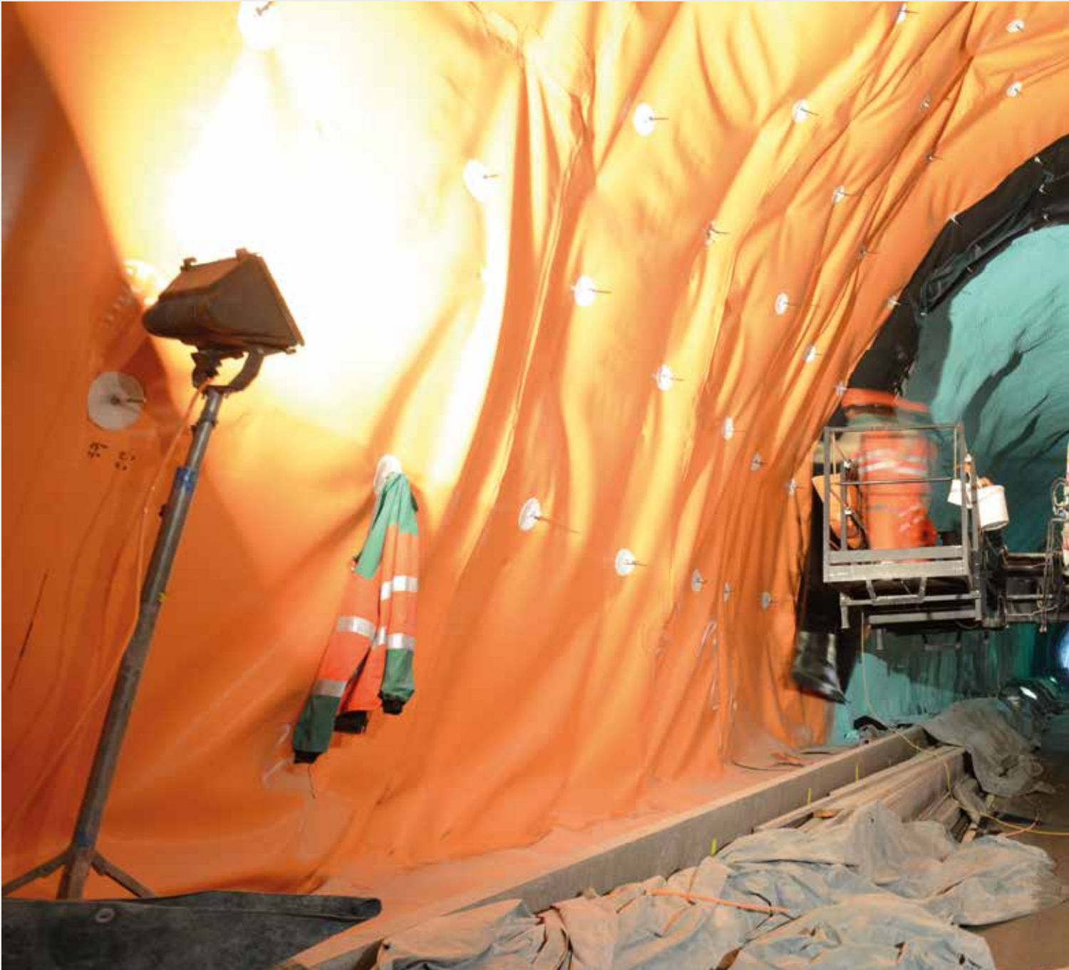
TUNNEL MITHOLZ, LÖTSCHBERG BASIS TUNNEL - Transition between MAPELASTIC TU SYSTEM spray applied membrane and MAPEPLAN synthetic waterproofing membrane
