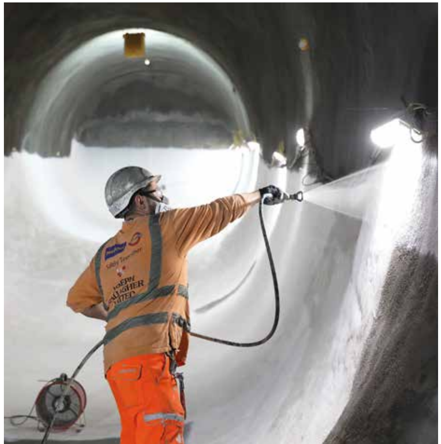
Application phases (gun fan direction)
