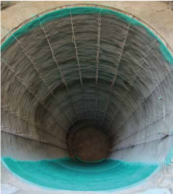
Example of re-bars installation
