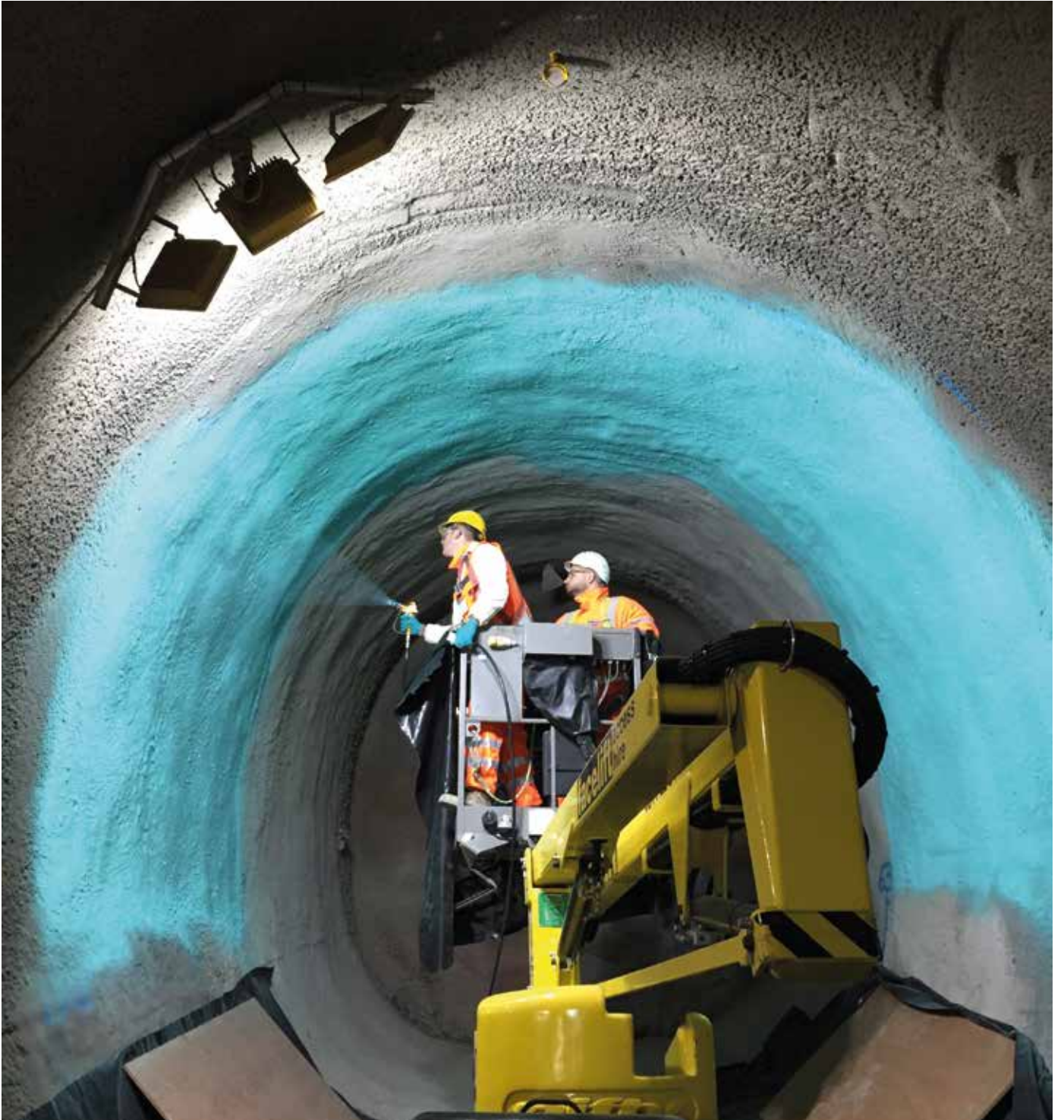
Application phase (distance from the substrate)
