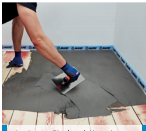
Application Planipatch Xtra + Latex Plus sur supports bois
