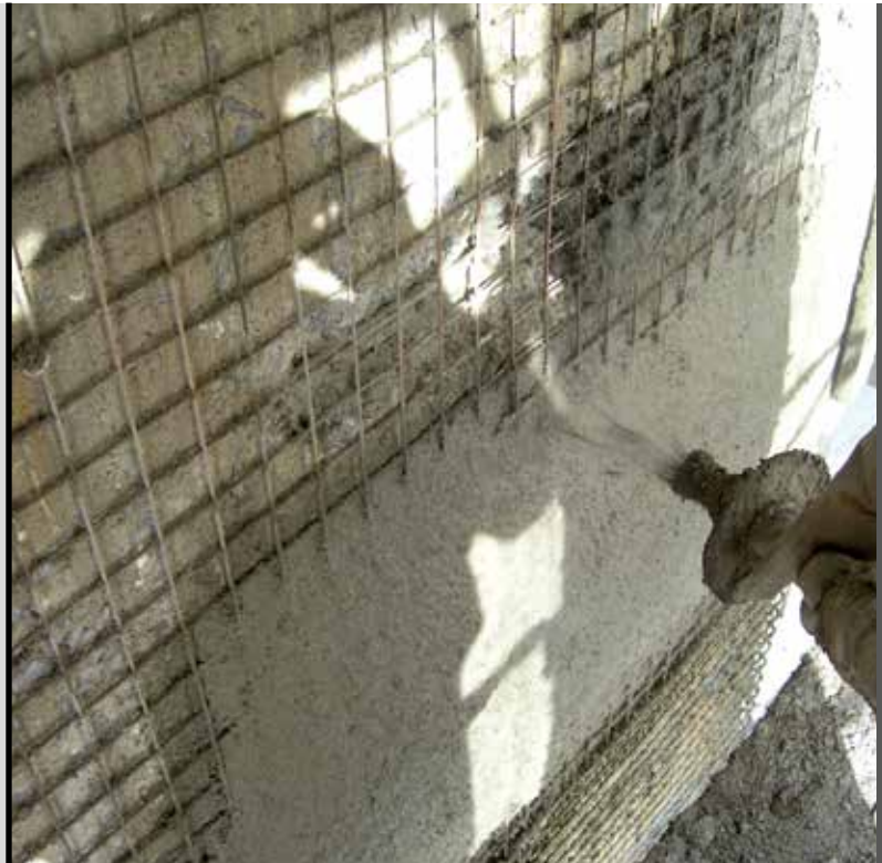
photo 7 MAPEGROUT BM applied by spray
