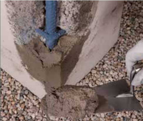
photo 9 Application of MAPEGROUT LM2K
