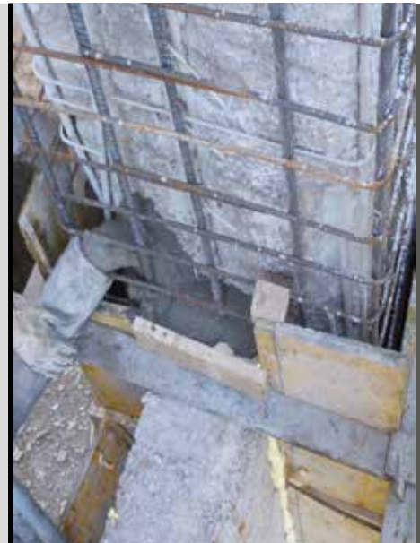
photo 12 Application of MAPEGROUT GF BETONCINO B1
