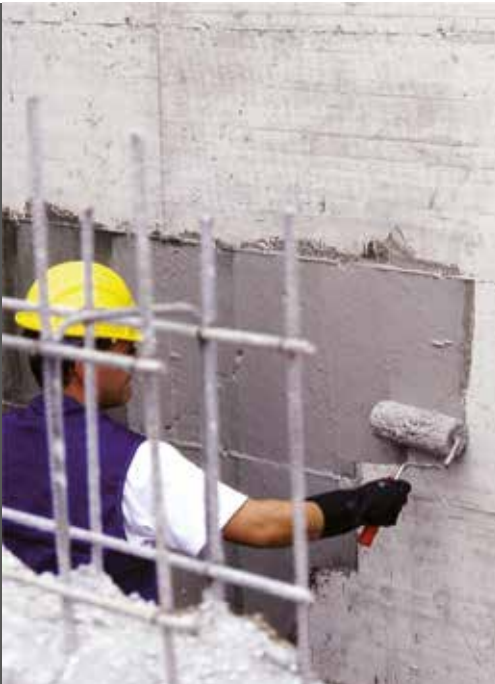
photo 17 MAPELASTIC SMART applied with a roller
