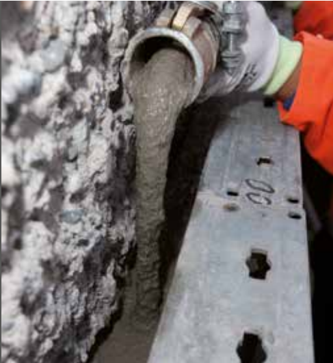
photo 11 Application of MAPEGROUT HI-FLOW GF
