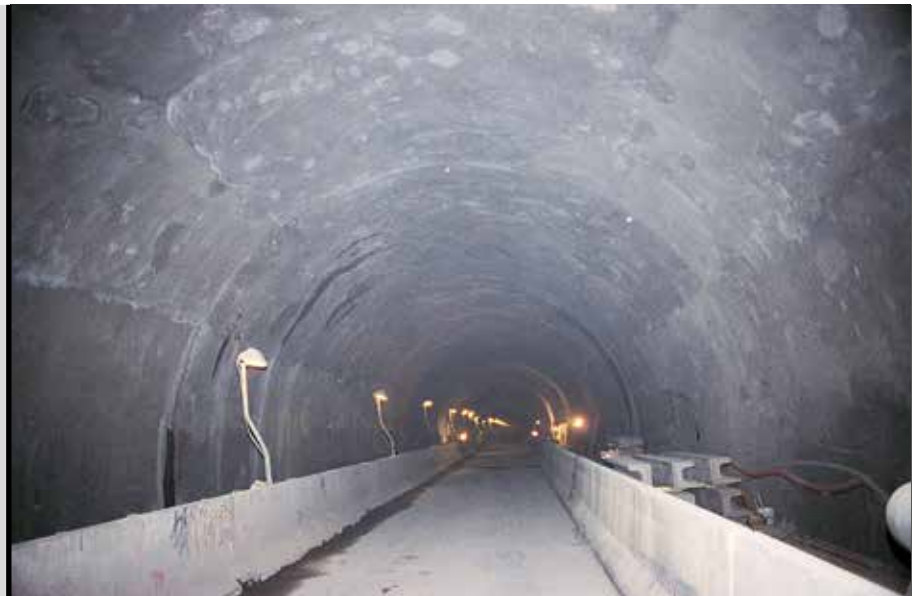
photo 6 Structure repaired using MAPEGROUT T60
