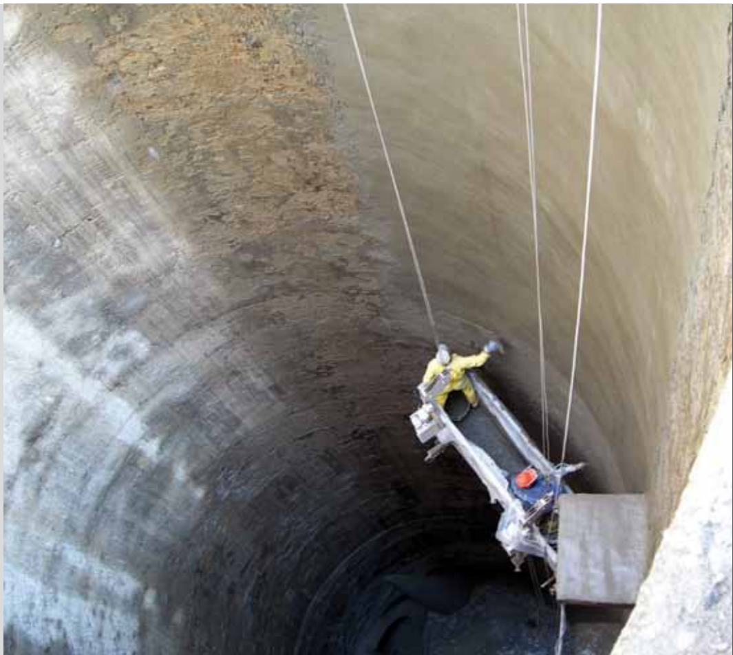
photo 6 Structure repaired using Mapegrout T60
