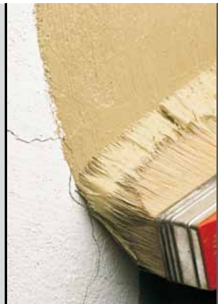
photo 19 Application of Elastocolor Paint
