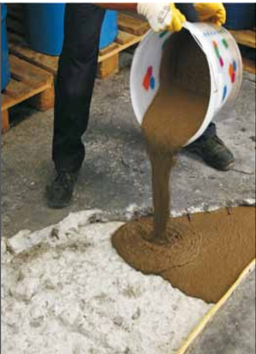
photo 12 Repairs to a floor using Mapegrout SV Fiber
