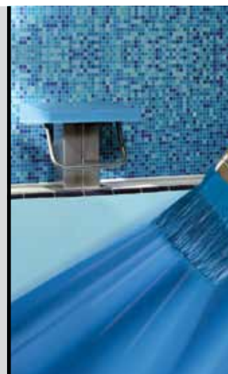
photo 20 Application of Elastocolor Waterproof
