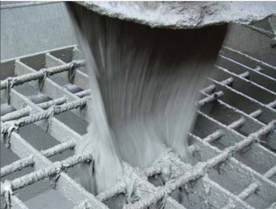
photo 14 Super-fluid concrete prepared using Stabilcem SCC
