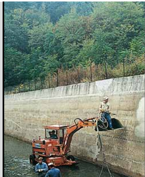
photo 18 Application of Idrosilex Pronto
