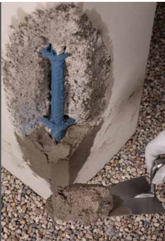
photo 10 Application of MAPEGROUT LM2K
