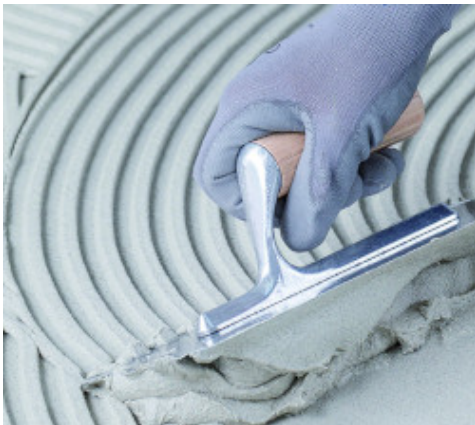
Spreading Adesilex P9 white
