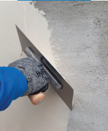
Application of PoroMap Finitura Civile on cured render
