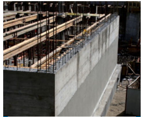
Retaining wall waterproofed after casting using Mapelastic Foundation
